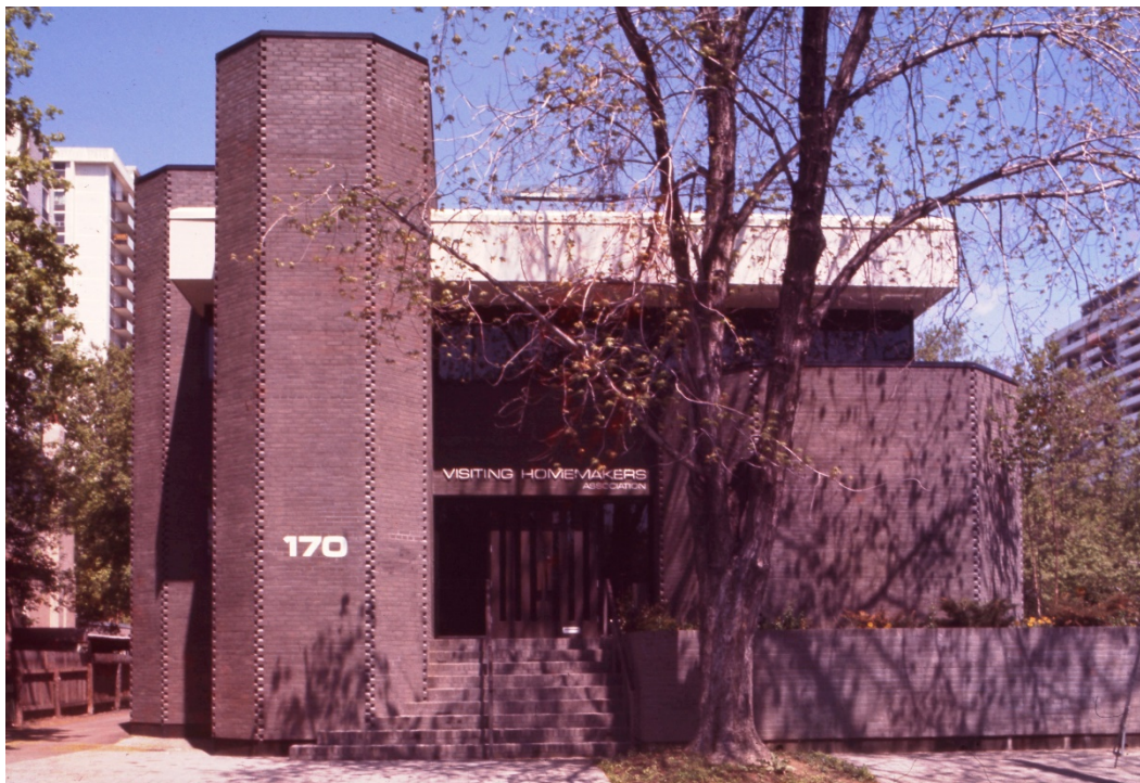
Early photograph of the VHA building showing the original pigment of the concrete brick cladding and paving (Leslie Rebanks)
