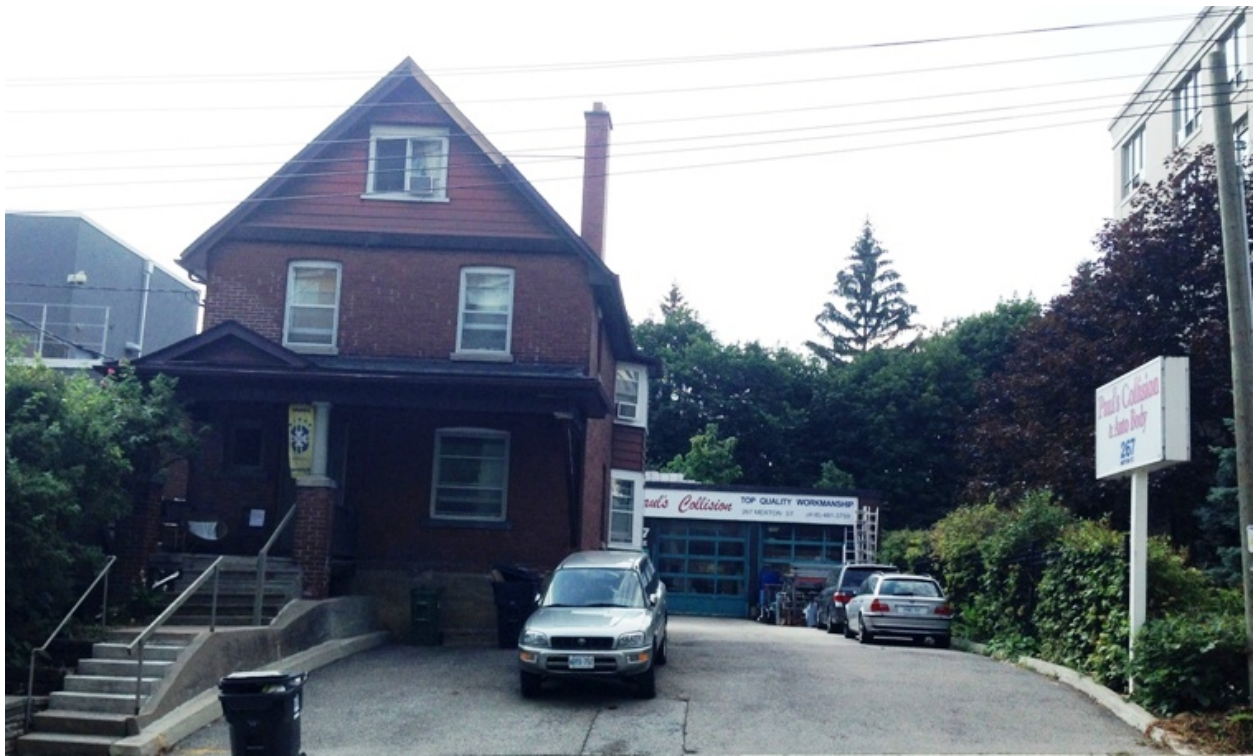
16. 267 Merton Street, south side of Merton Street, showing one of the remaining houses from the late 19th-early 20th century period with a later industrial use introduced behind the house. (HPS, 2017)
