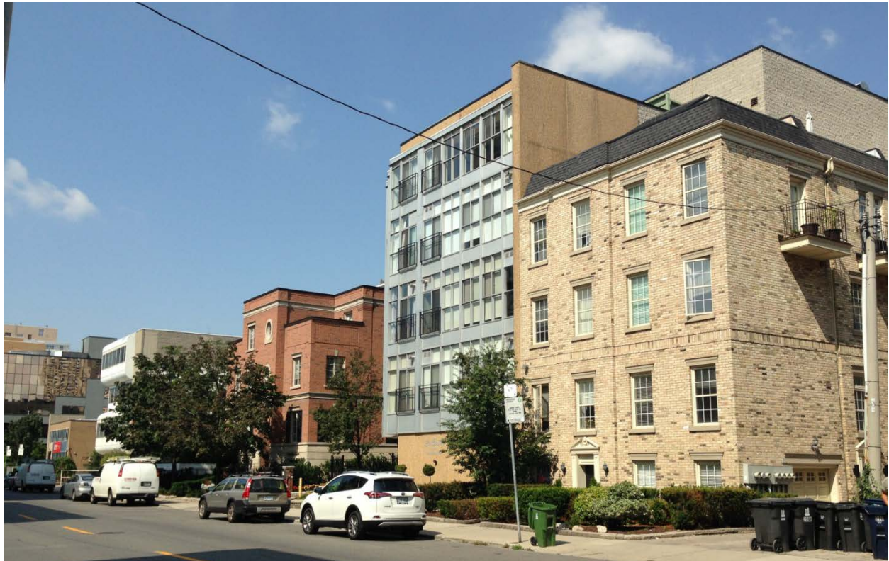
15. North side of Merton Street showing the context with recent low-rise townhouses and condominiums at 180, 194 and 200 Merton Street and beyond the tree which marks 170 Merton, the low-rise office building occupied by the Geneva Centre for Autism at 164 Merton Street (HPS, 2017)
