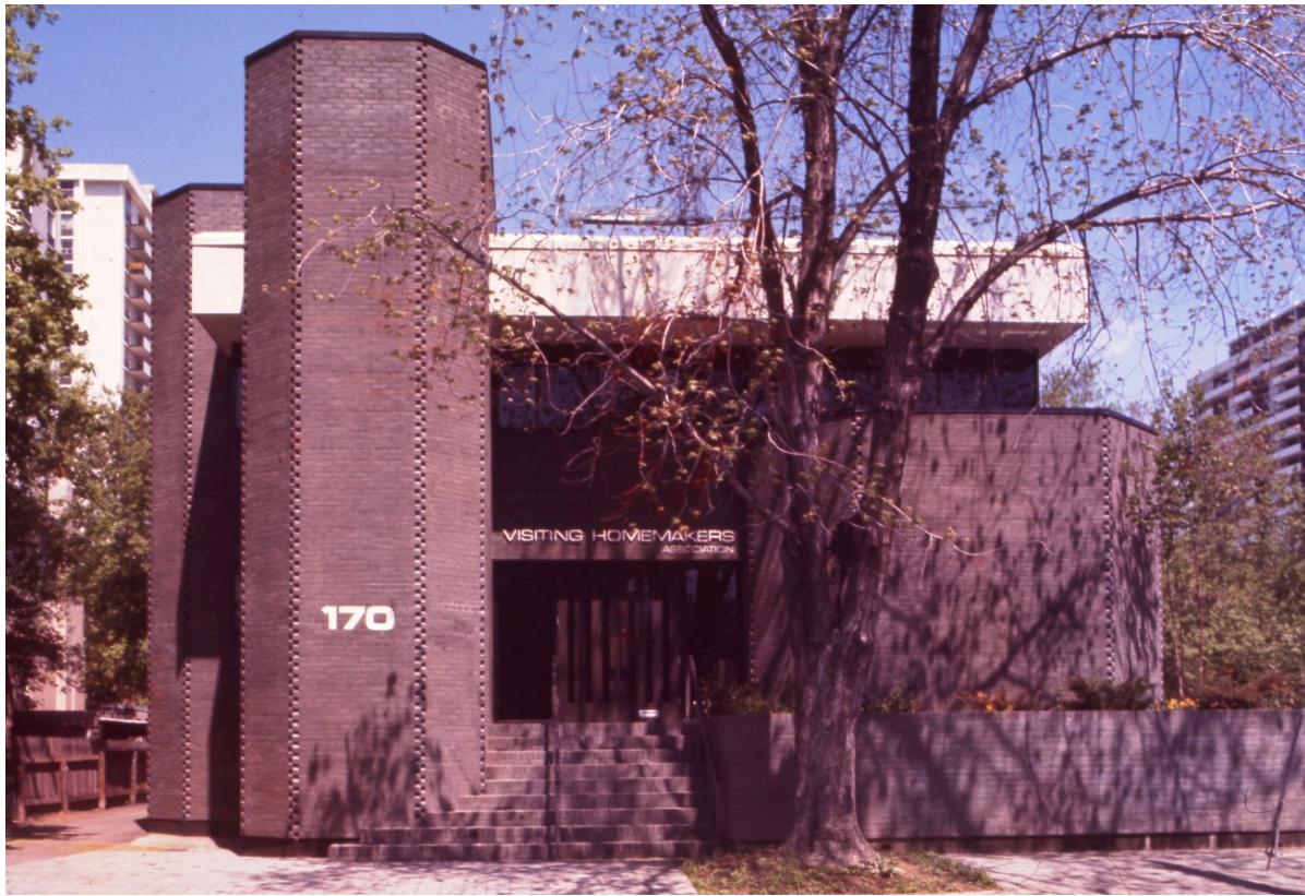
8. VHA, South Elevation showing an early photograph of the building with the original pigmented concrete brick and three of the towers with the entrance stairs and the planted terrace (Leslie Rebanks)
