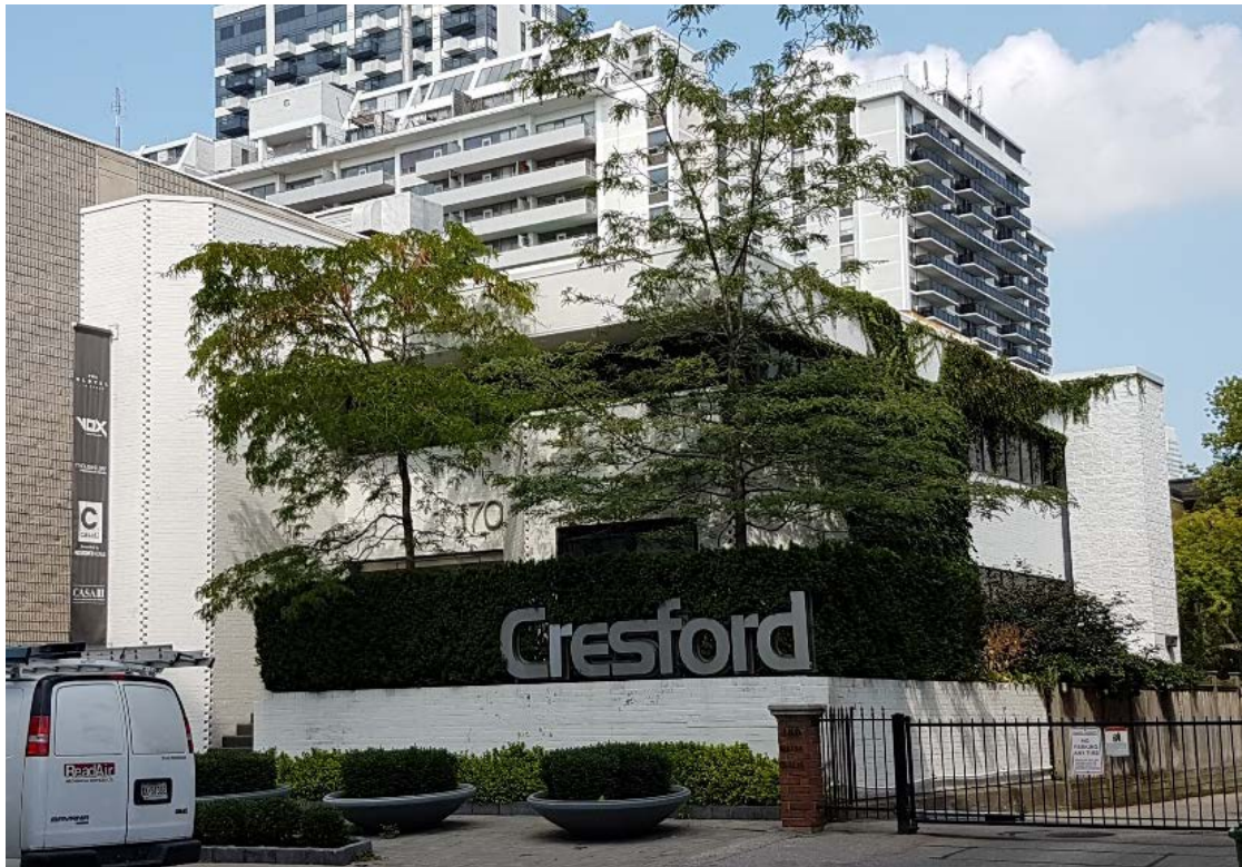
Photograph of the VHA building, principal (south) and side (east) elevations (HPS, 2017)
