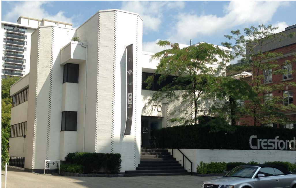
Photograph of the former Visiting Homemakers Association (VHA) building, currently occupied by Cresford Developments, 170 Merton Street, principal (south) and side (west) elevations (Heritage Preservation Services (HPS), 2017)
