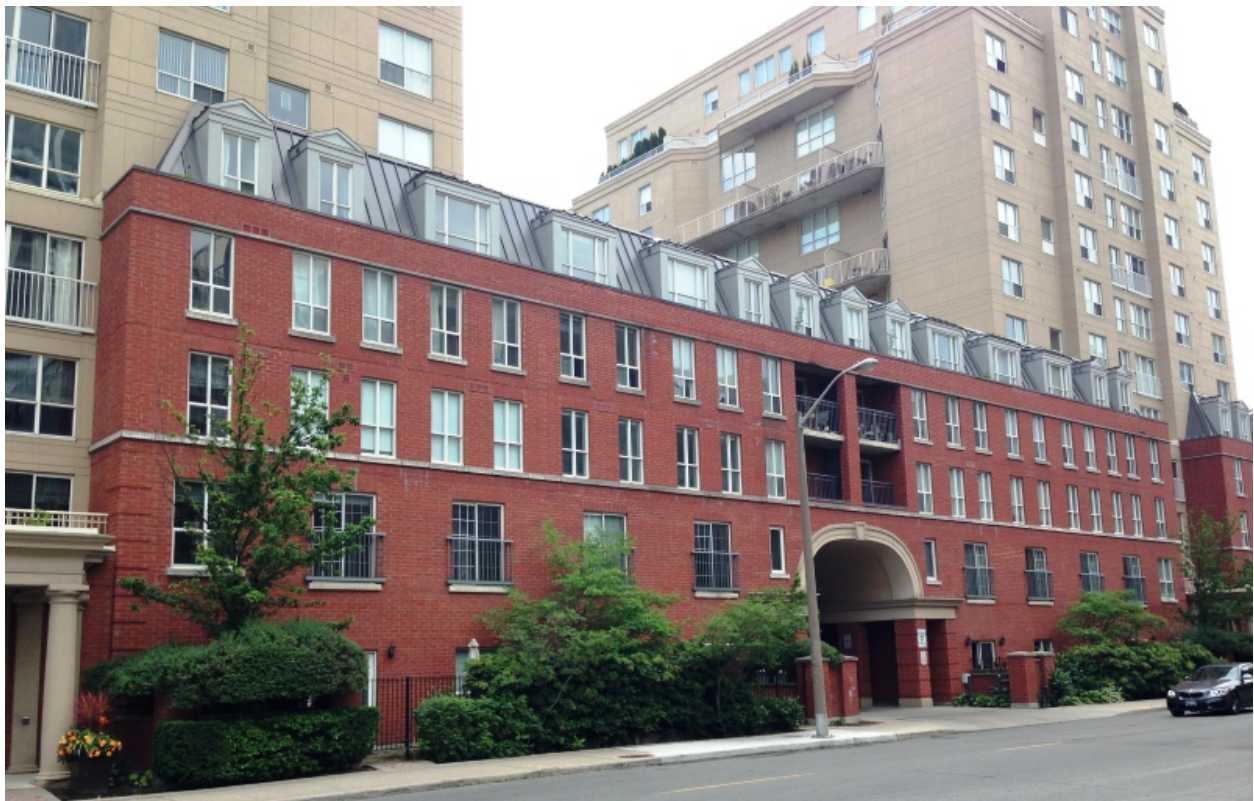
19. 119-139 Merton Street, mix of low-mid-rise housing at 119-139 Merton Street completed in 2001. (HPS, 2016)
