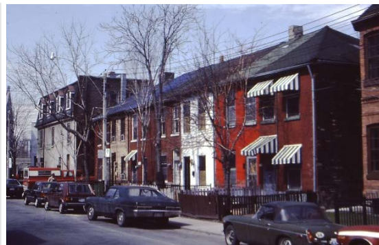
3f. Archival Photograph, 1982
