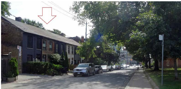
5c. Context looking south from King Street East with Little Trinity Church Precinct and Enoch Turner Schoolhouse on the right
