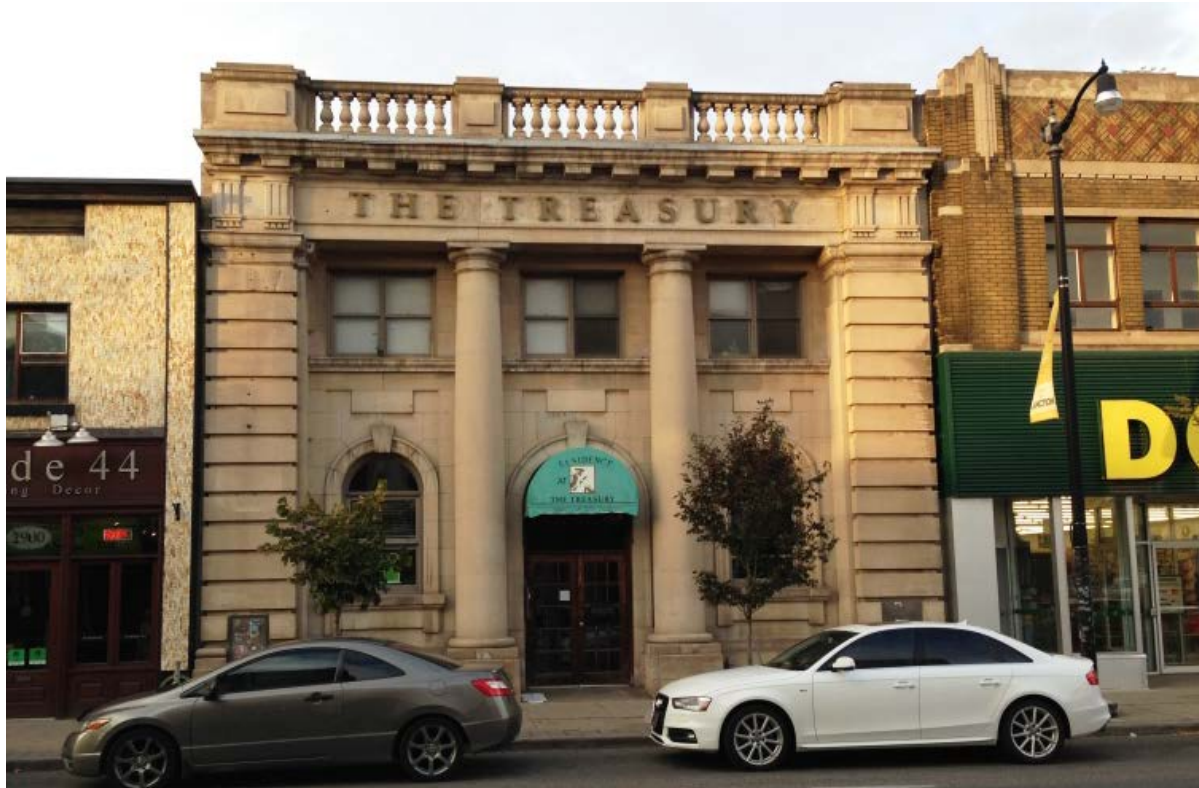
Photograph of 2896 Dundas Street West, principal (south) elevation. (Heritage Preservation Services [HPS], 2017)
