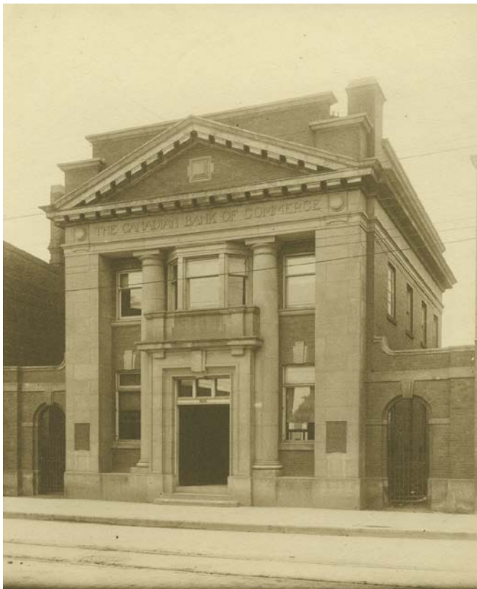
10. Canadian Bank of Commerce (1905-1909), Darling and Pearson Architects, 2886 Dundas Street West shortly after completion of construction. Demolished c.1935 (CIBC Archives)
