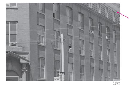
East elevation detail (1975) showing 4th storey windows originally had brick jack arches, not stone lintels 1936
