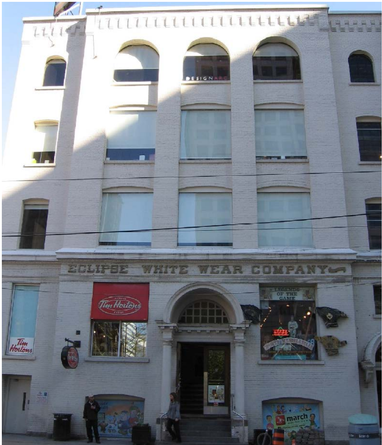
322 King Street West - Eclipse Building
