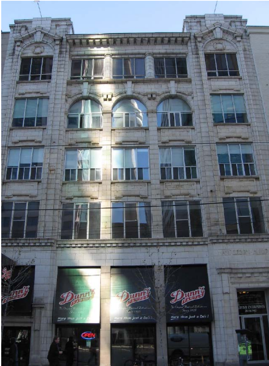
284 King Street West - Anderson Building
