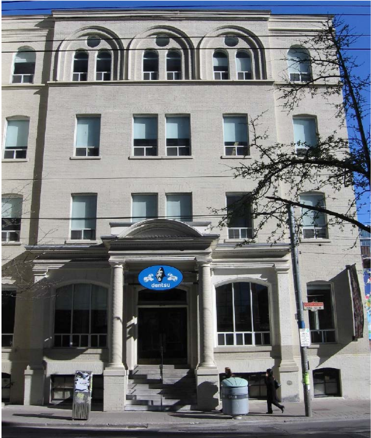
276 King Street West - Reid Building (to be demolished)
