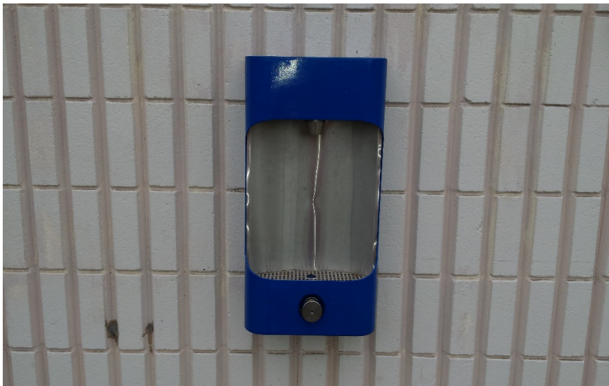
Figure 2: Water Bottle Filler Installed at a Park Building Adjacent to Multiple Amenities
