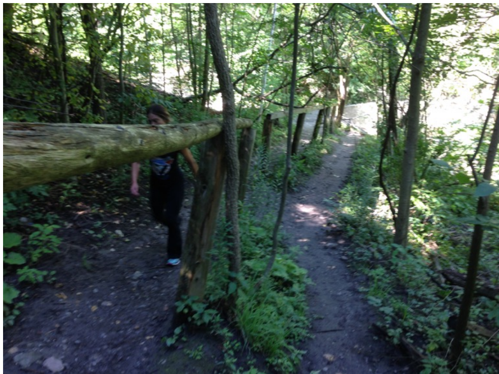
Path up to Shaftesbury steps (formal path to left of partially missing railing)
