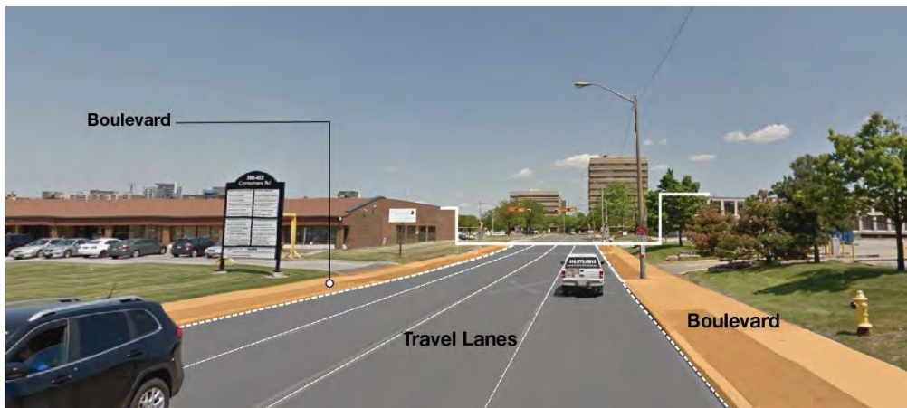
Exhibit 4-19: Existing Streetscape Character on Consumers Road
