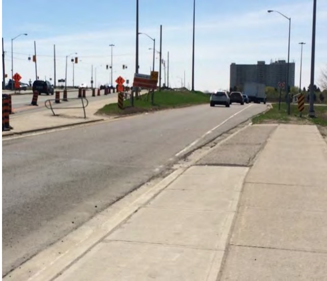
Exhibit 4-38: Victoria Park Avenue on-ramp at Highway 401 WB – lack of pedestrian crossing markings
