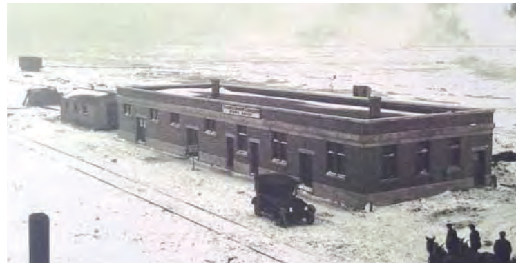
Harbour Commissioners Building
