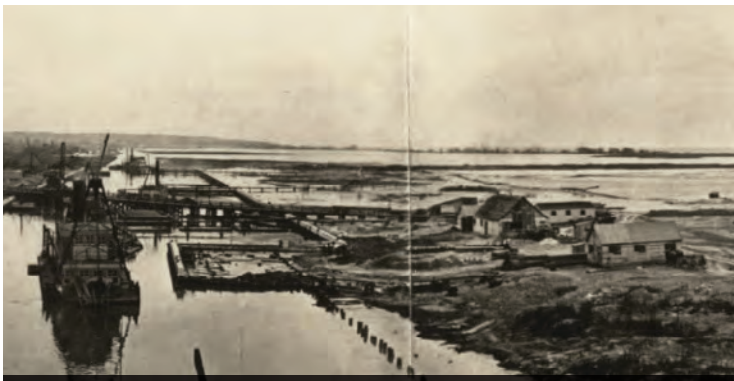
1914 View s.e. showing Keating Channel, the Harbour Commission Workshop and Office, and Queen’s City Foundry
