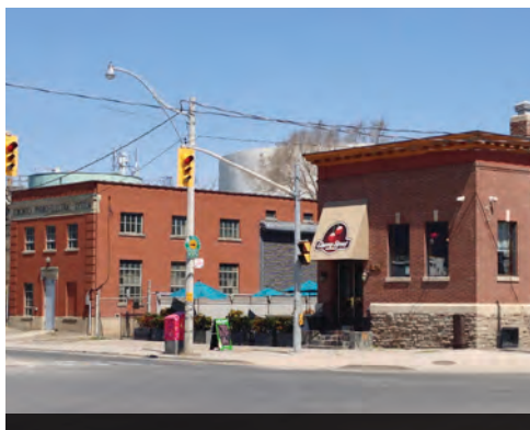
Toronto Hydro Substation and the Dominion Bank Building
