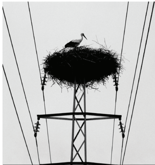
Stork nest on a transmission tower
