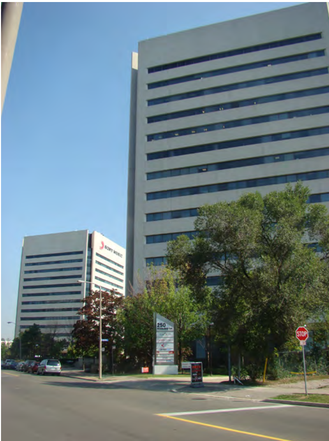
Figure 56: Office buildings south of Eglinton Avenue East.
