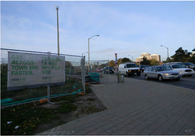
Figure 73: Crosstown LRT construction staging at Don Mills and Eglinton
