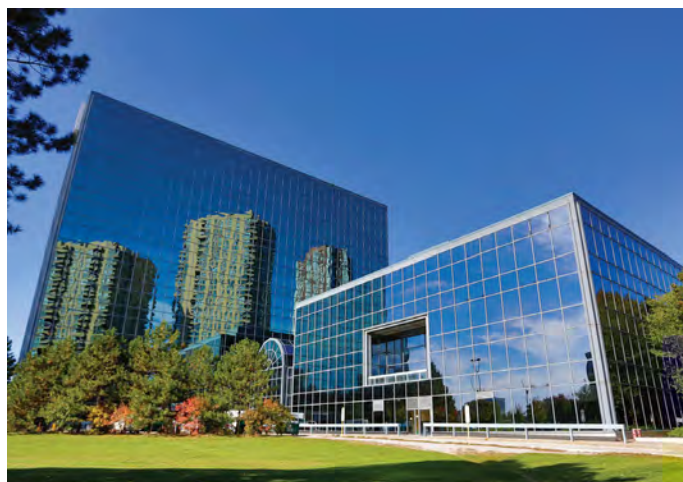
Figure 35: Employment buildings at 1 and 3 Concorde Place (Google Images, 2016)
