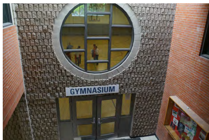
Figure 60: Gymnasium at Dennis R. Timbrell Resource Centre
