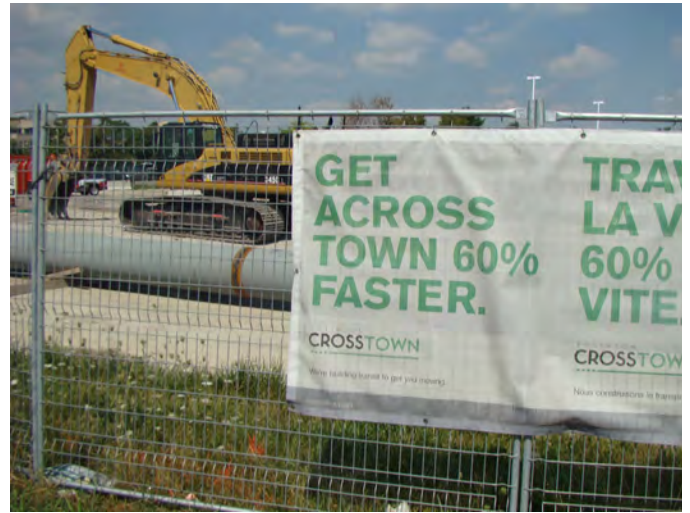
Figure 47: Construction staging for Crosstown LRT
