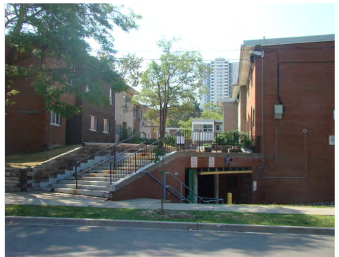
Figure 33: Low scale built form in Flemington Park built above parking structures exhibiting poor grading relationships with the street
