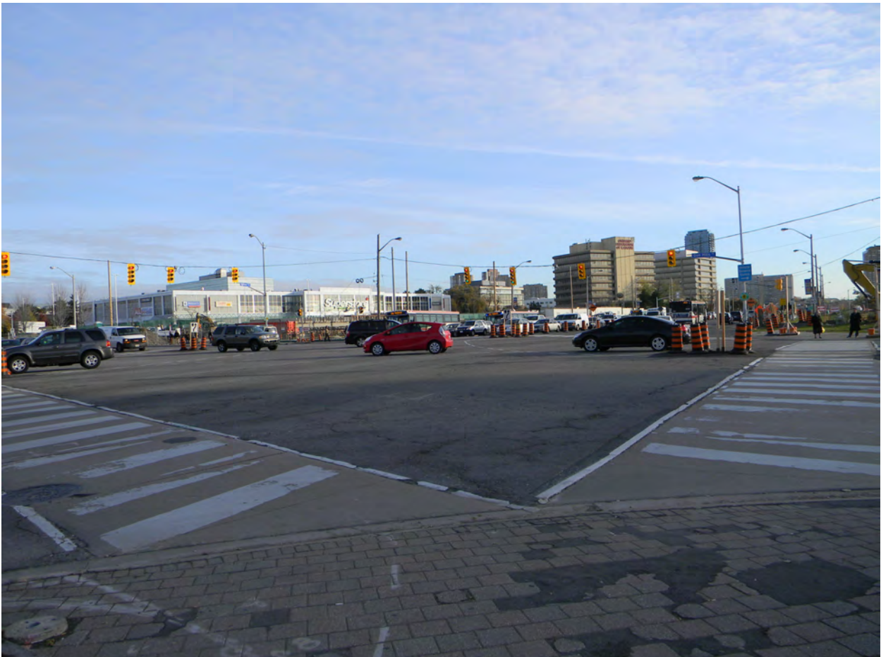
Figure 45: Intersection of Don Mills Road and Eglinton Avenue East
