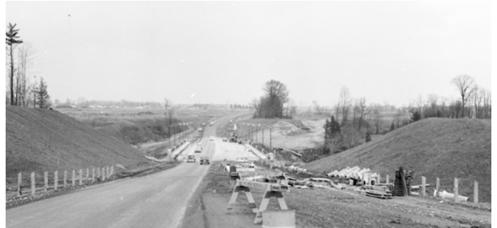
Figure 1: Eglinton Avenue East under construction, looking east, near East Don River. (1956)
