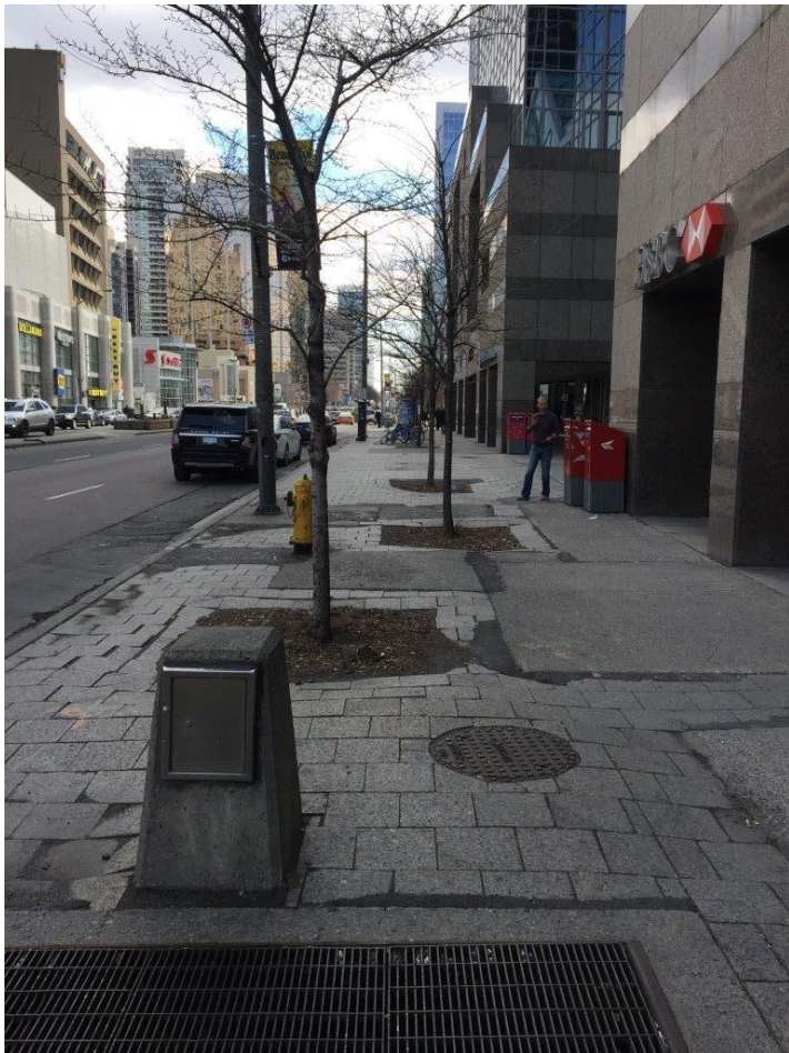
Figure 1 - The Current Streetscape Condition is in Disrepair
