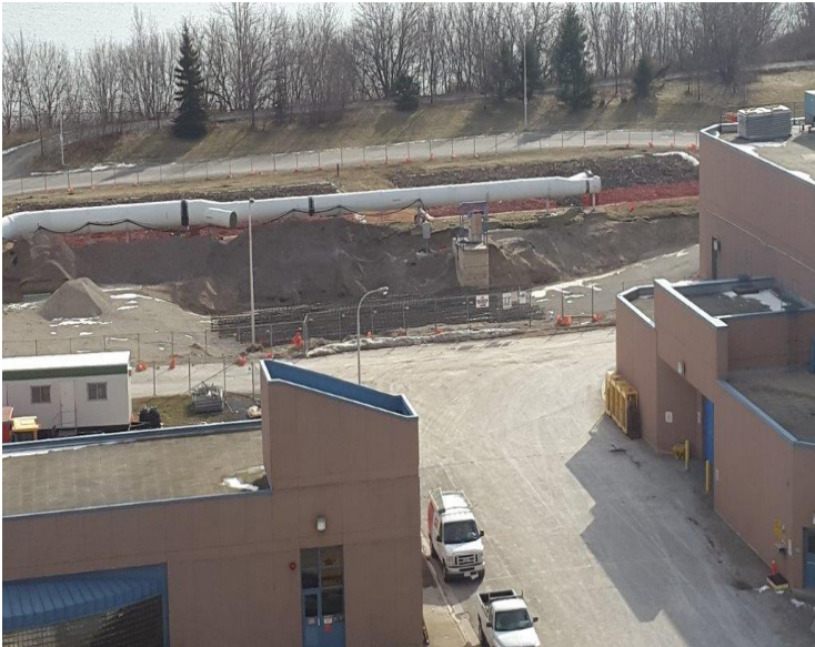
c) Foul Air Inlet Piping Installation
