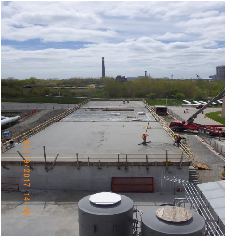
b) Roof Top Membrane on Biofilter Building
