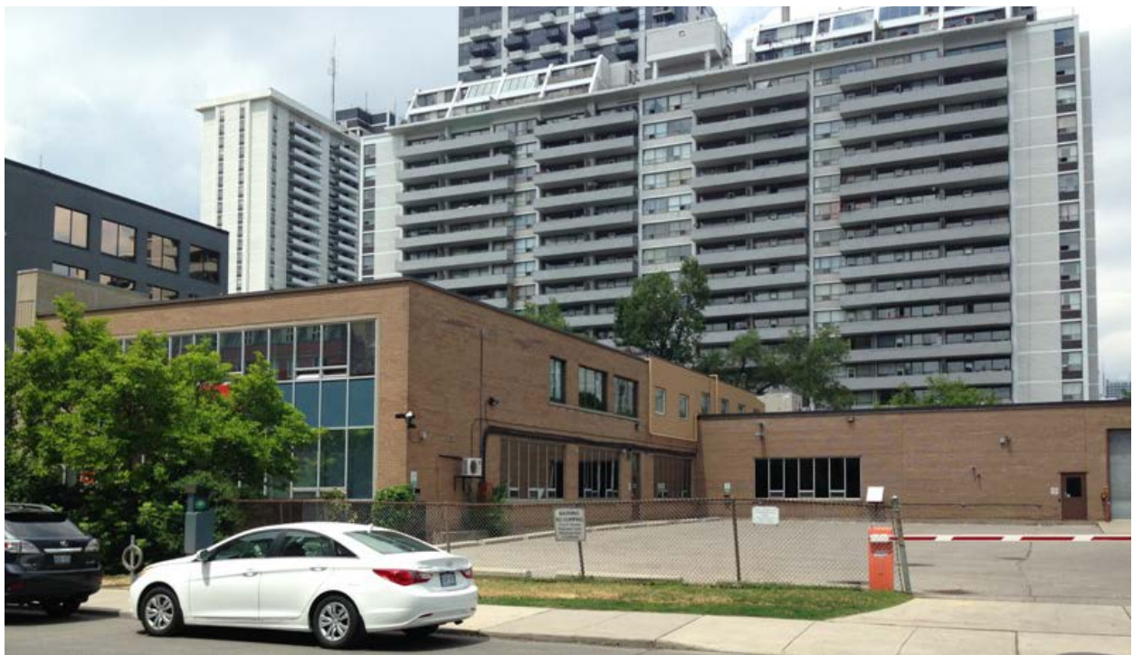
11. 140 Merton Street: photograph showing the principal (south) elevation and the east side of the property. Note at the rear of the original building, the second-storey addition constructed in 1985 indicated by the different coloured brick, as well as the single-storey addition, at the rear of the parking lot completed in 1973. (HPS, 2016)
