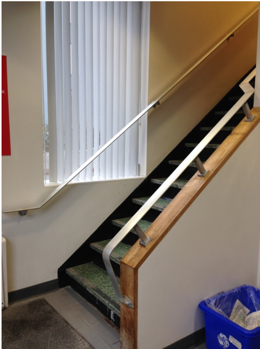
24. Entry Stairs in lobby adjacent to elevator showing: green terrazzo treads and balustrade trimmed in wood with a handrail similar to the exterior stairs (HPS, 2017)
