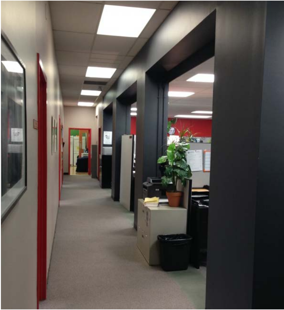
17. Interior on the east side of the second floor showing the original external wall (at the right) of the narrower upper floor prior to the extension (centre and left) in 1985.
