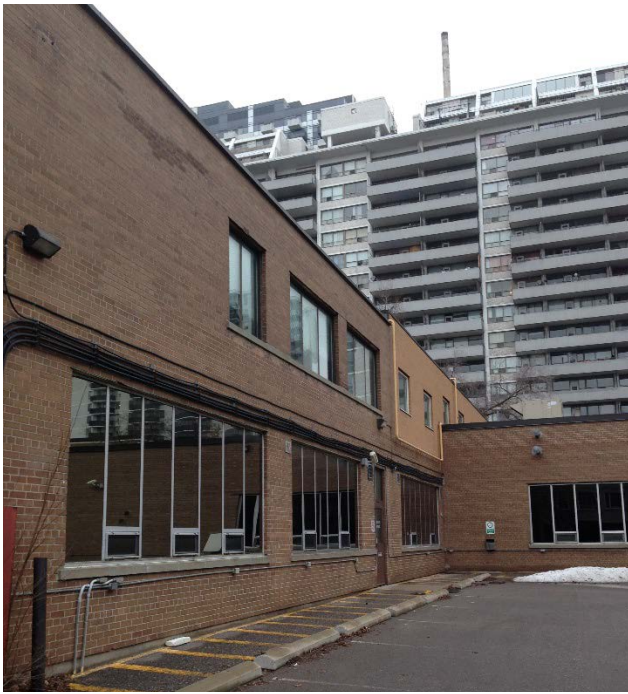
15. East elevation showing the office windows (left). The ground floor windows were likely replaced in 1973 as they match those of the warehouse extension (to the right). The pattern of mullions and lower opening sections corresponds to the front, south elevation, curtain wall. The windows at both levels, while maintaining the original pattern are new glazing systems (HPS, 2017)
