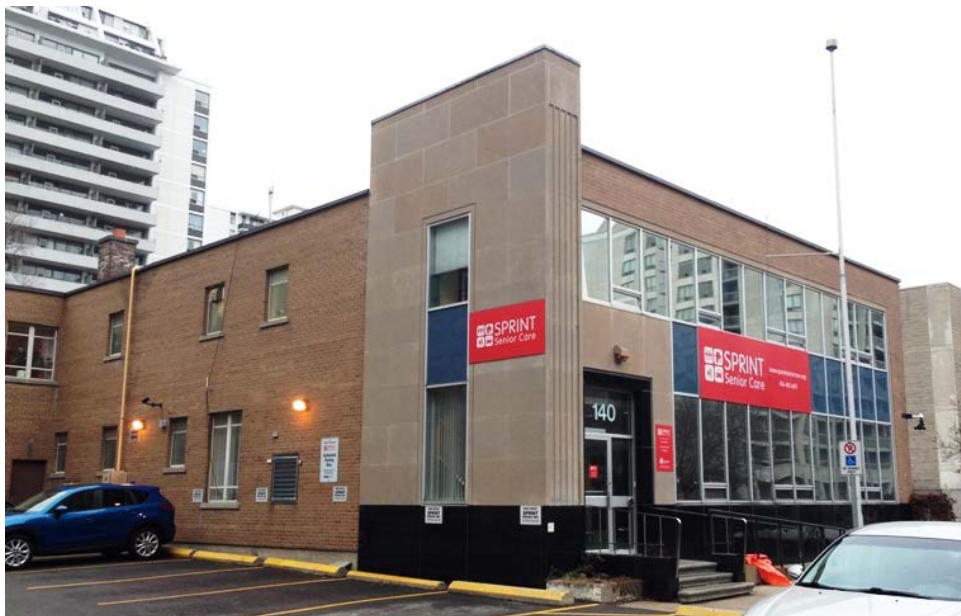
16. Side (west) and principal (south) elevations: showing the west elevation with its steel windows for a ground floor office and washrooms (smaller). The ground floor window, and that viewed in the upper corner represent typical glazing system of the east, west and north elevations with opening systems at the top and bottom of the window to provide a variety of options to enhance comfort and cross ventilation. (HPS, 2017)
