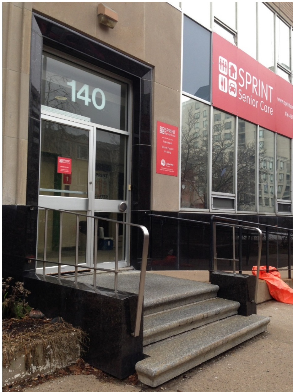
21. Entry at 140 Merton Street, viewed from the west: showing the granite steps flanked by polished black granite base for the balustrade and the door frame with later ramp handrails to the right in black hollow metal tubing and the curtain wall details with the opening sections (HPS, 2017)
