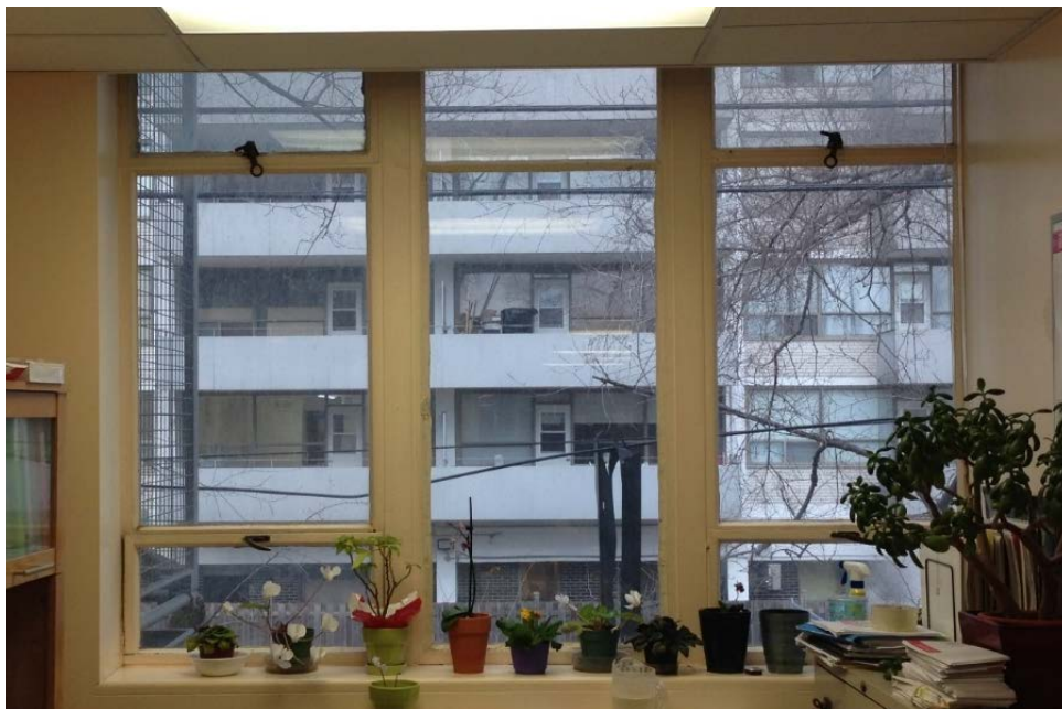
23. Interior views of typical steel section windows with brass openers (HPS, 2017)
