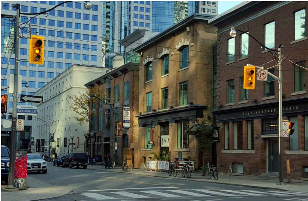
16. Current Photographs, 14 Duncan Street, 2016: looking north from Duncan Street to Adelaide Street West (above) and south from Adelaide to King Street West (below) and showing the Telfer Paper Box Building's location on the northwest corner of Duncan and Pearl streets (Heritage Preservation Services).
