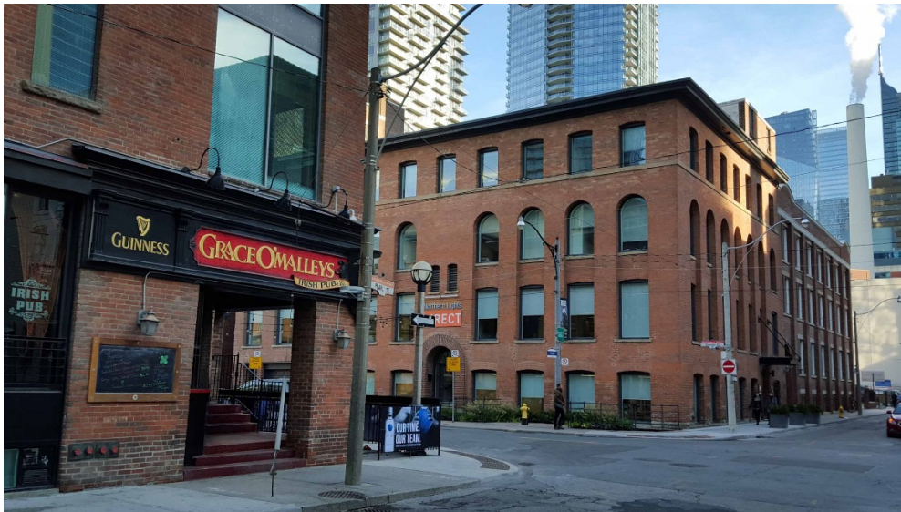
17. Current Photographs, 14 Duncan Street, 2016: showing the south elevation on Pearl Street (above) with the 1902 building and part of the 1906 addition, and the entrance at the southeast corner (below) with the Canada Printing Company Building and the White Swans Mills Building in the background (Heritage Preservation Services).
