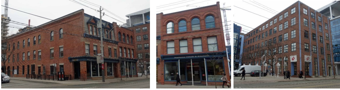
7a, 7b & 7c. 254 King (left), 256 King (centre), and 266 King, South Building (right)
