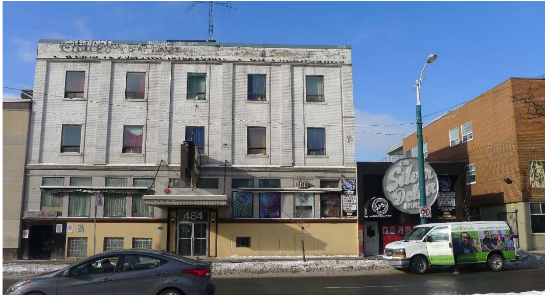
Principal (east) façades of 484 Spadina Avenue, the Waverley Hotel and the Silver Dollar Room (Heritage Preservation Services, February 2014)
