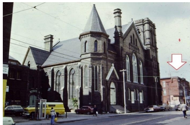
2f. Archival Photograph, 1977
