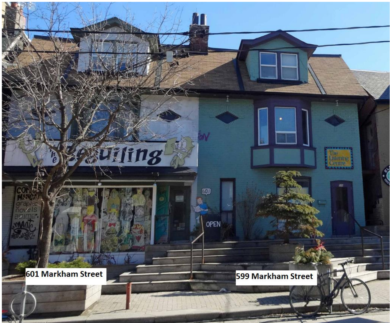
599-601 Markham Street: showing the west (principal) elevations (HPS, 2015)
