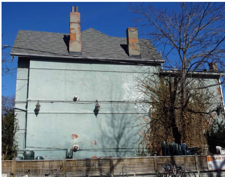
581 Markham Street: showing the south elevation at the north-east corner of Markham and Lennox Streets (HPS, 2015)
