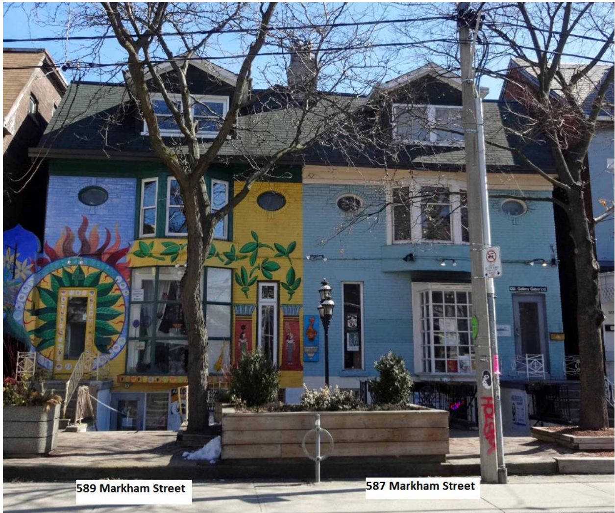
587 - 589 Markham Street: showing the west (principal) elevation (HPS, 2015)
