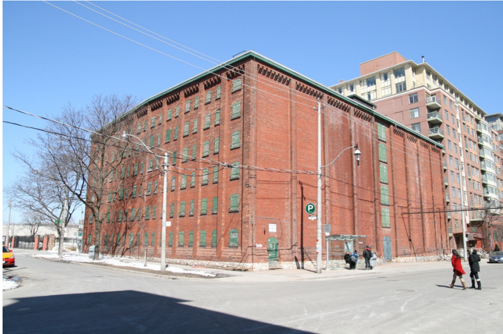
View from South-West Looking North East
