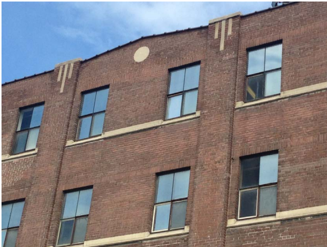
23. Principal, south elevation showing the stone details including the particular cut of the window sills, the vertical bands on the pilasters with their stone caps, the pediment with its stone disc and the vertical soldier courses above the window heads stretching from pilaster to pilaster (HPS, 2017)
