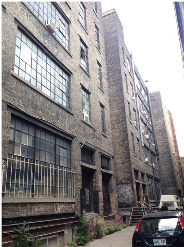
South elevation, Purman Building (HPS, 2017)
