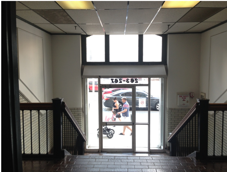
26. Entry Lobby showing the original metal and wood handrail and the glazed brick tile dado. (HPS, 2017)
