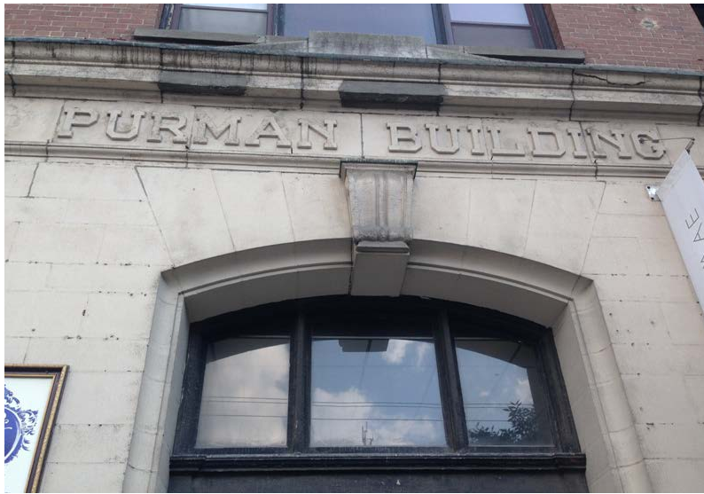
20. Detail of top of main entry with the Purman Building name, the arch with corbel keystone and the small pediment above the cornice. (HPS, 2017)
