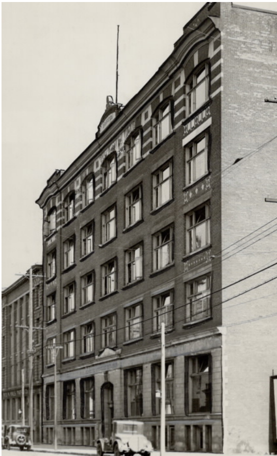
16. Photograph of the Purman Building taken in 1928 showing the original cornice details. (TPL, tspsa_0112898f)
