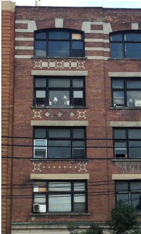
21. Decorative brick and stone panels which are featured at the outer bays of the building (HPS, 2017)
