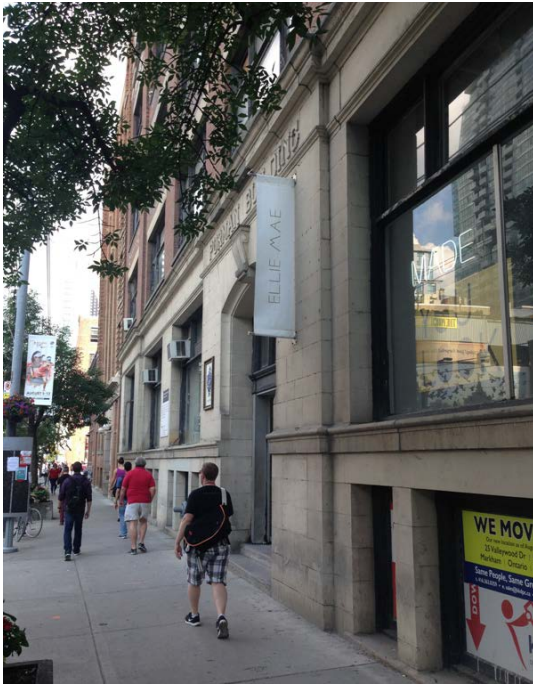
18. View of the base of the Purman Building (HPS, 2017)
