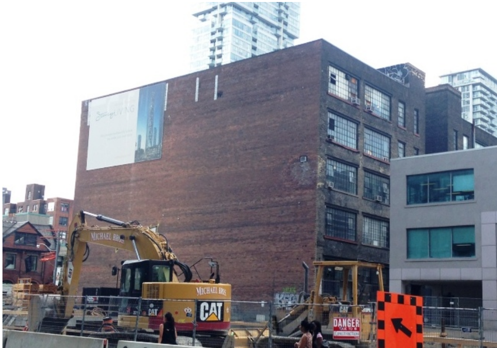
Photograph of the west and south elevations, Purman Building. (HPS, 2017)
