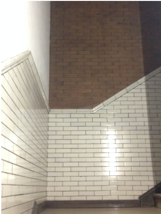
27. Main Stairs showing the glazed tile dado and brick walls above. (HPS, 2017)
