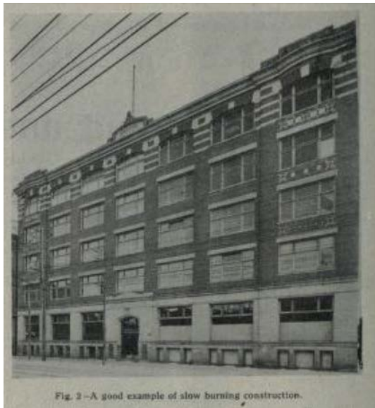
10. The Purman Building, "a good example of slow burning construction" featured in Denison's article for Contract Record, March 1917, p. 220.
