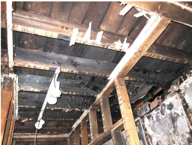
The third floor of 303 George Street (The Frank Beecroft Houses) showing evidence of fire damage
