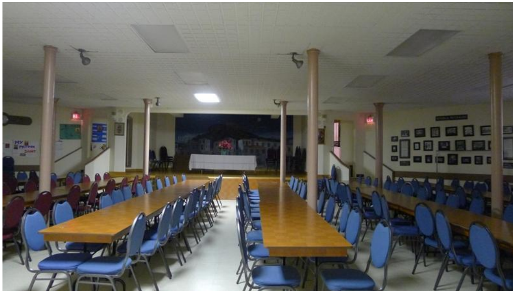
30. 115 Bond Street, Basement: showing the octagonal space of the basement with its metal column supports, looking east towards the stage (HPS, 2016)
