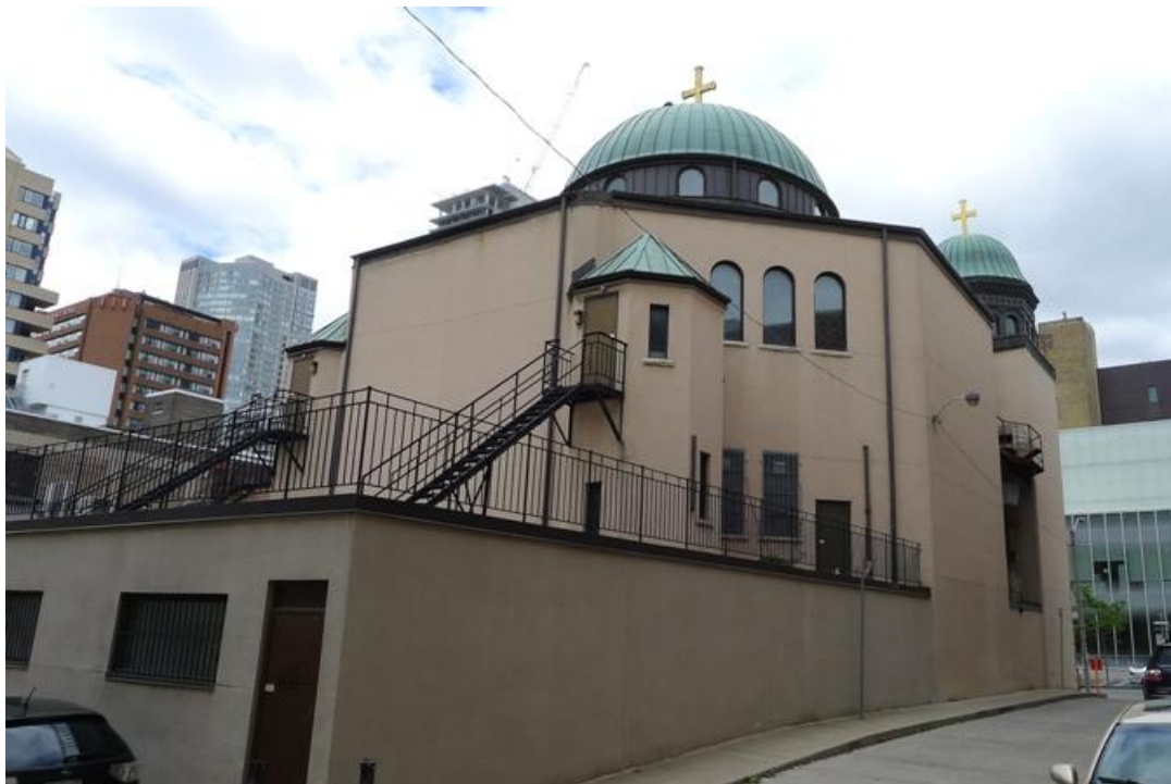
19. 115 Bond Street: showing the rear north and east elevations, the principal octagonal volume of the domed prayer space, the two small towers for the spiral stairs and the 1958 one-storey extension. (HPS, 2016)
