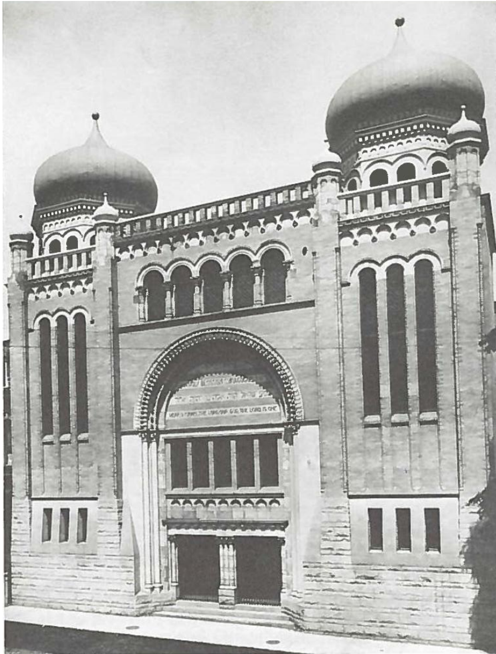
Holy Blossom Synagogue (now St. George's Greek Orthodox Church), 115 Bond Street, showing the original 1895-7 west elevation facing Bond Street as originally designed as a synagogue. (Arthur, 1986)
