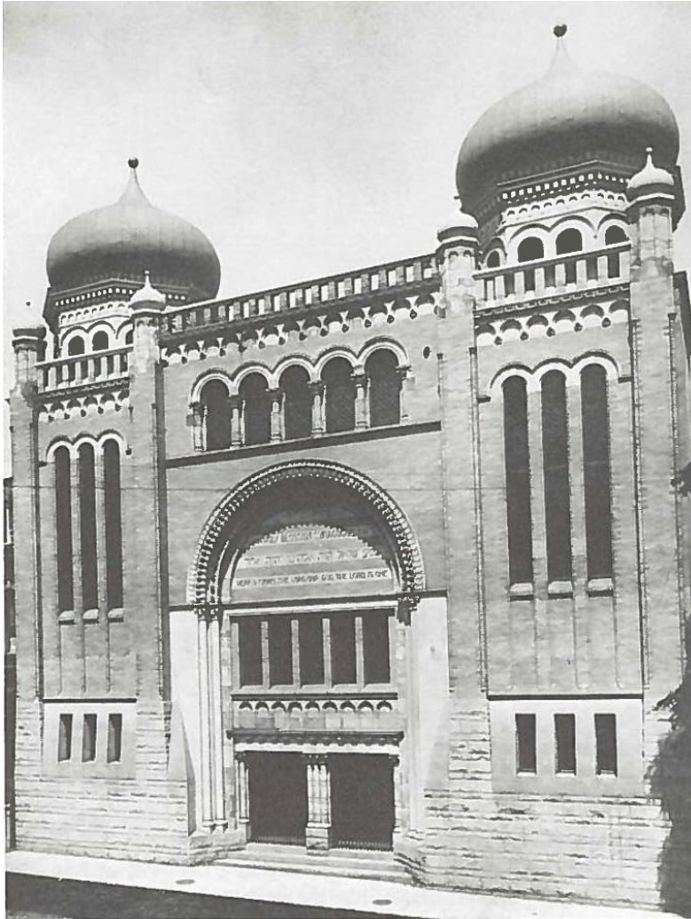
SAINT GEORGE'S GREEK ORTHODOX CHURCH (FORMER HOLY BLOSSOM SYNAGOGUE) 115 BOND STREET, TORONTO
