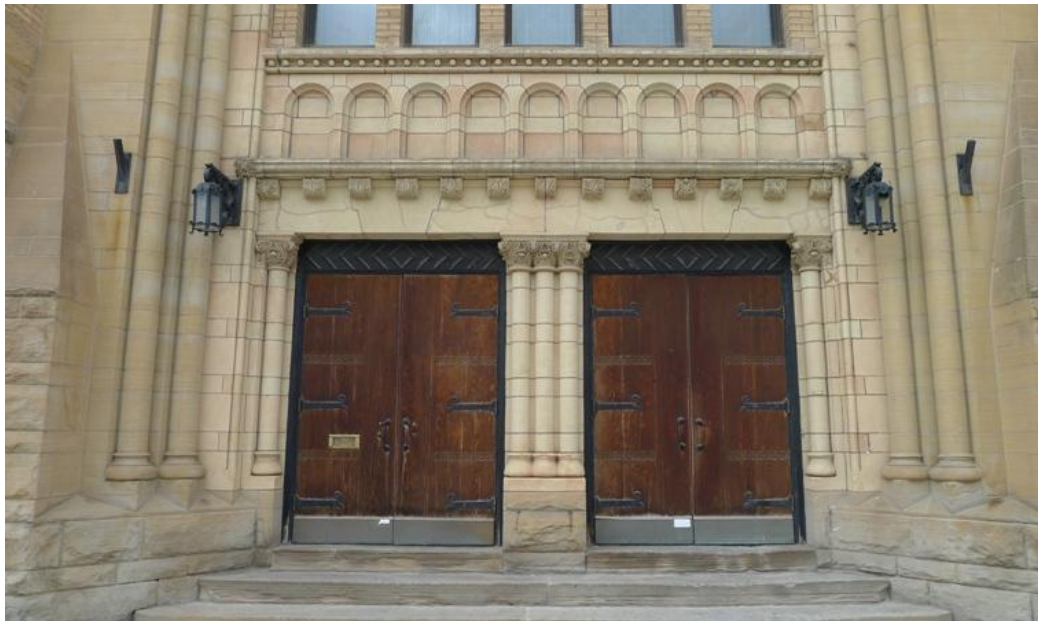
22. 115 Bond Street: showing the west elevation and the decorative details including the colonettes, capitals, decorative brackets, and the arcade. Note particularly how the alternating pattern of narrow and deep stone height is integrated into the elements of the façade. (HPS, 2016)
