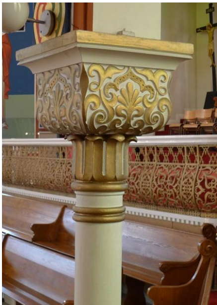
34. 115 Bond Street, Capital: showing one of four original capitals supporting the pendentives of the great central dome whose design is derived from the Courtyard of the Lions, at the Alhambra, Spain. (HPS, 2016)
