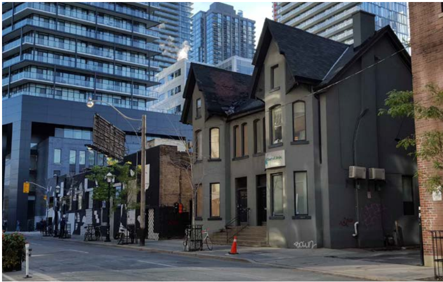
15. Current Photograph, 357 and 359 Richmond Street West, 2016: the principal (north) elevations of the houses are shown (left), as well as the west wall of 359 Richmond (right), which overlooks the laneway separating it from the 401 Richmond complex (Heritage Preservation Services).
