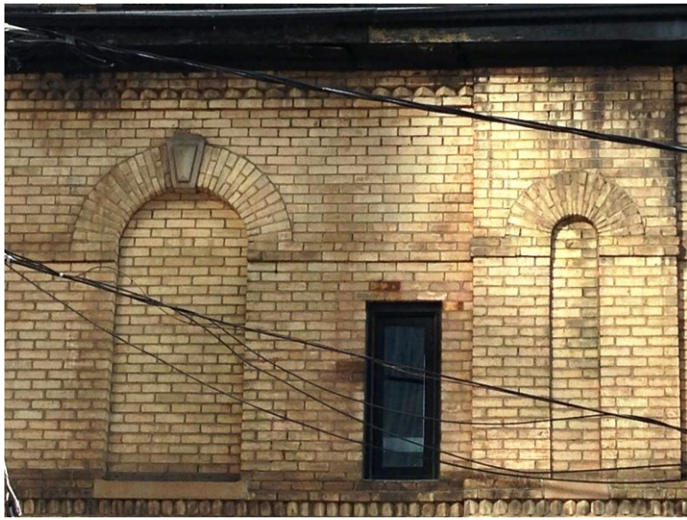
29. 79 Shuter Street, West elevation: showing the decorative brick work, the saw tooth courses, string courses and blind panels as well as the cast stone keystone. (HPS, 2016)
