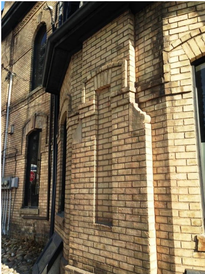
30. 79 Shuter Street, west elevation: showing the brick details, string courses, and the stone keystones, relief panels and chimney mouldings. (HPS, 2016)
