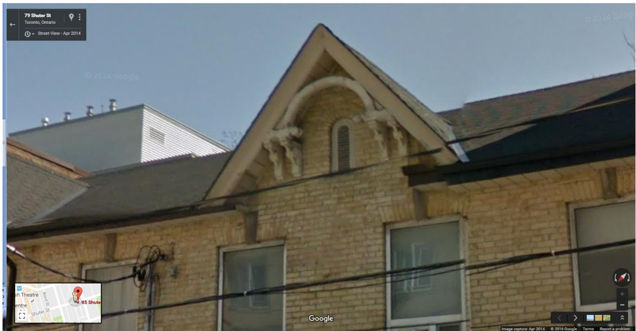
24.81 Shuter Street, North elevation, gable details. (Google Street view, April 2014)
