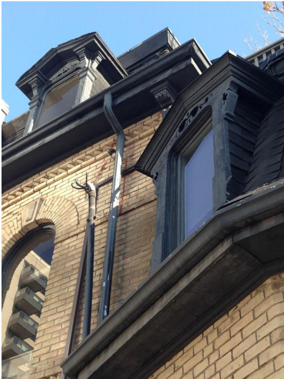
31. 79 Shuter Street, west elevation: showing the details in the mansard dormer window casings as well as the brick details. (HPS, 2016)
