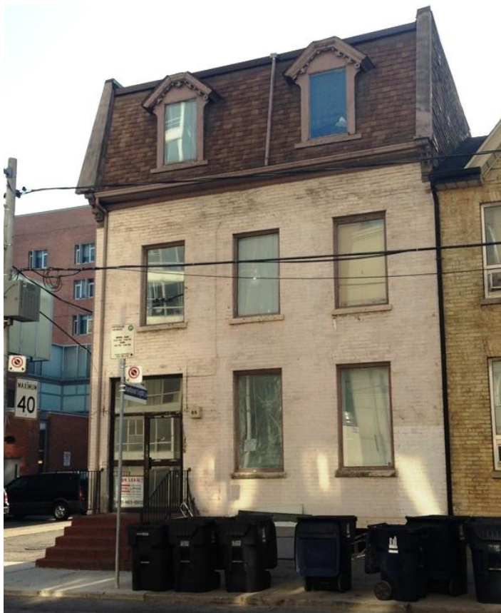
85 Shuter Street, showing the north elevation (HPS, 2016)
