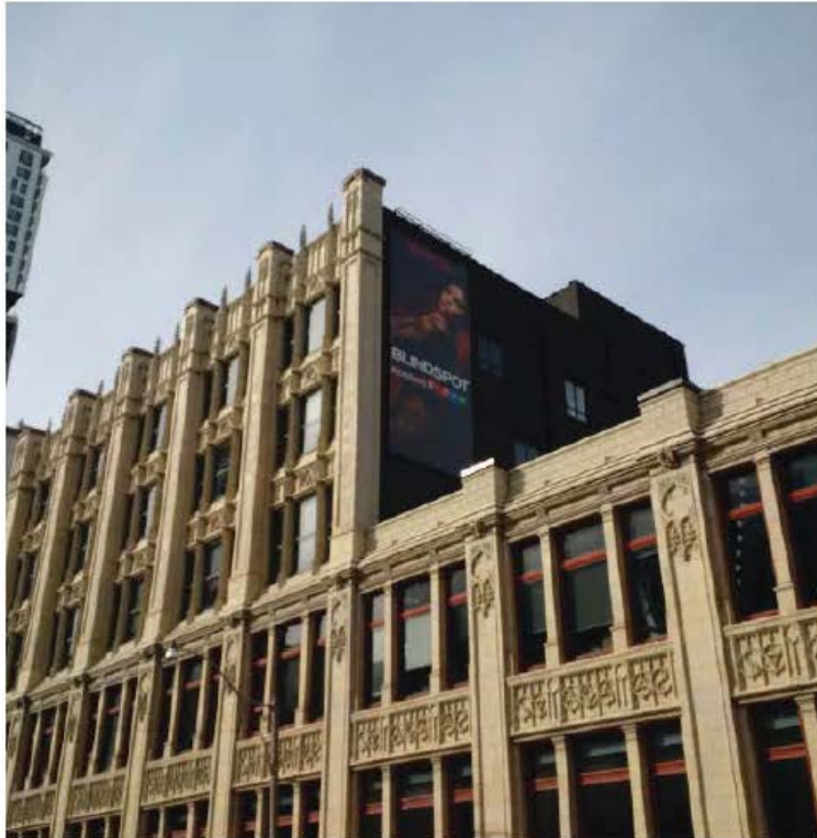
Figure 9: First party sidewall signage on the upper floors of the designated heritage building at 250 Queen Street West, Present Day.
