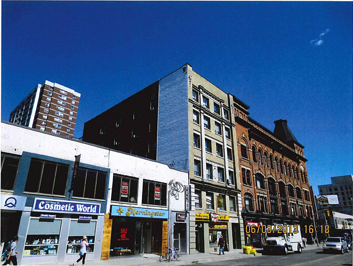
Figure 8: Blank sidewall following removal of mural at 615-617 Yonge Street.
