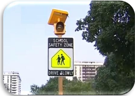
Flashing Beacon with Timer
