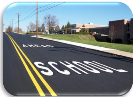
School Stencil Pavement Markings Speed Markings
