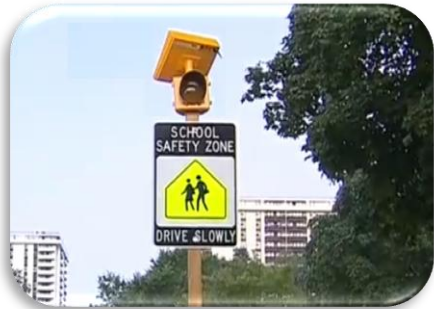
Flashing Beacon with Timer
