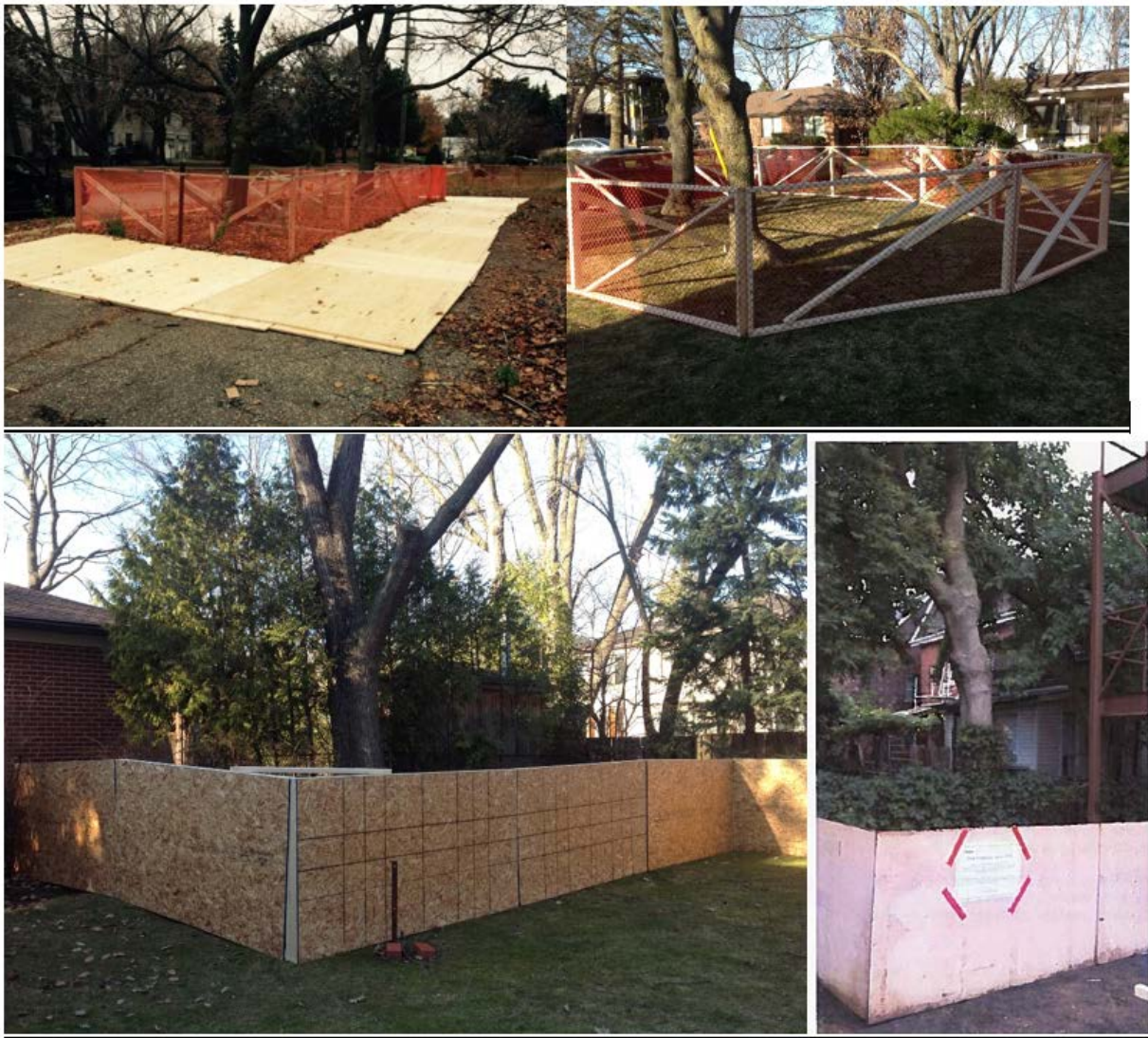
Photo 1: Examples of Different Types of Tree Protection Measures
