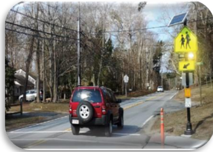
New Rapid Flashing Beacons at Crosswalks (Optional)
