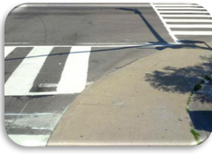
Enhanced Pedestrian Crosswalk Markings
