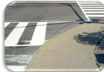
Enhanced Pedestrian Crosswalk Markings
