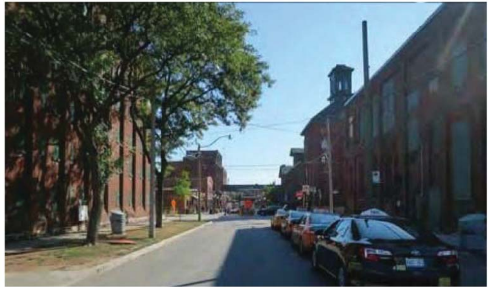
VIEW 4 EXISTING PHOTOGRAPH - N.T.S.
