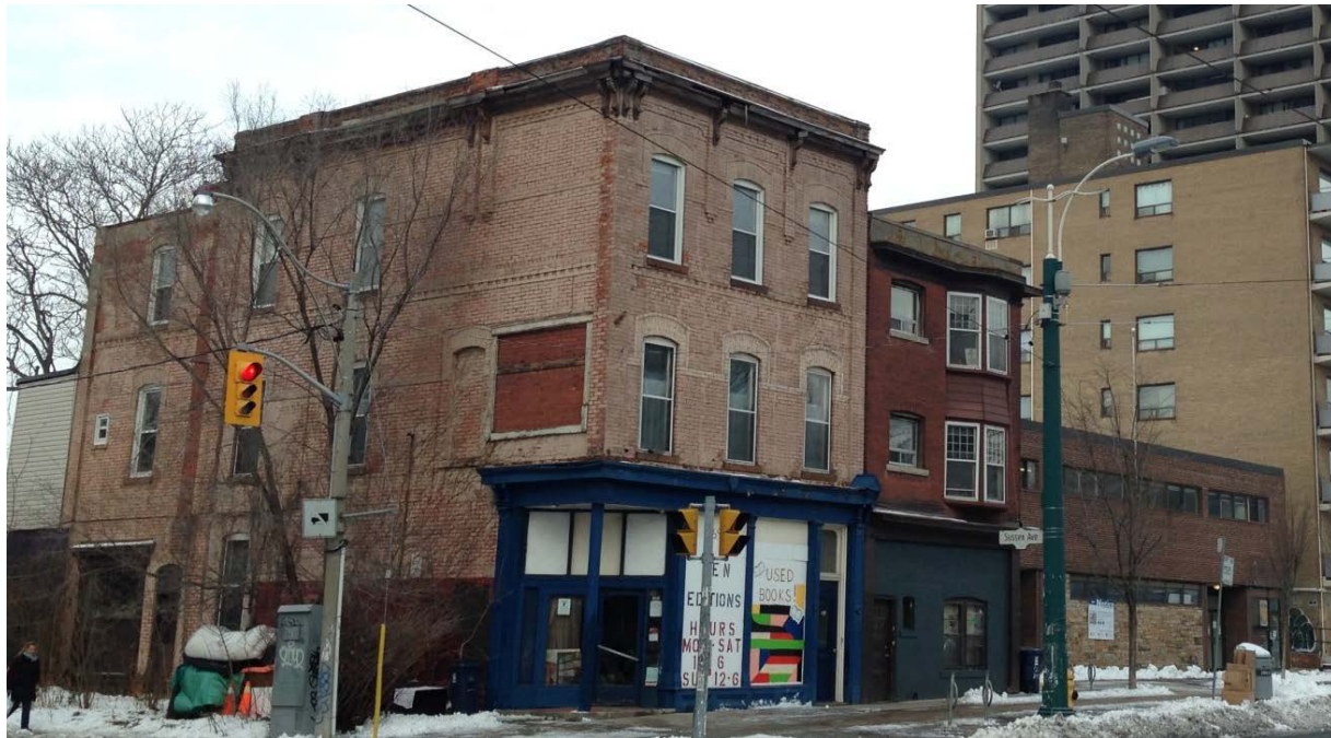
Photograph of 698 Spadina Avenue showing its principal elevation facing east towards Spadina Avenue and side elevation facing south to Sussex Avenue.
