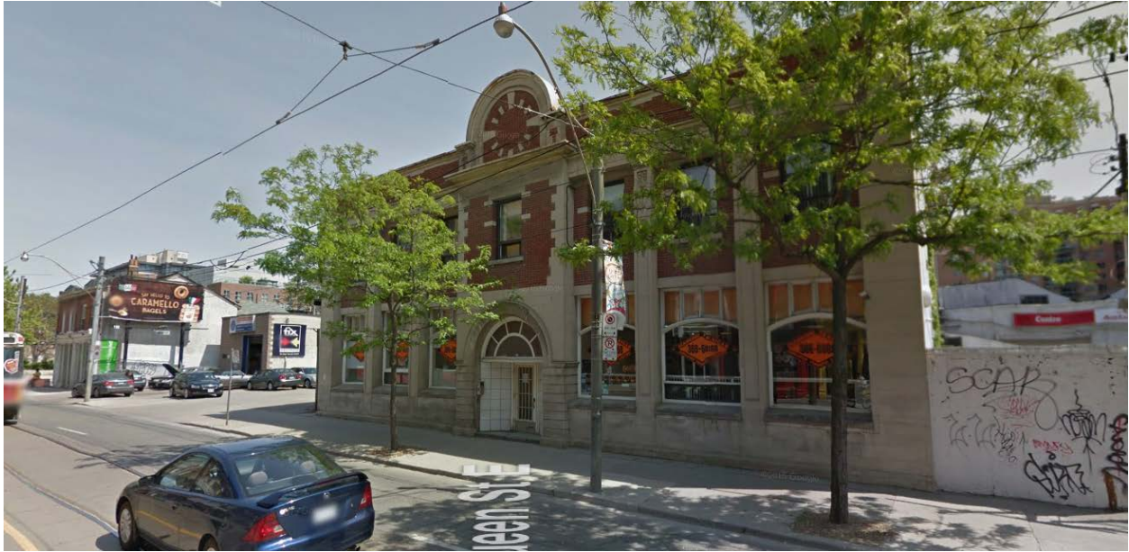
245 Queen Street East - North Elevation
