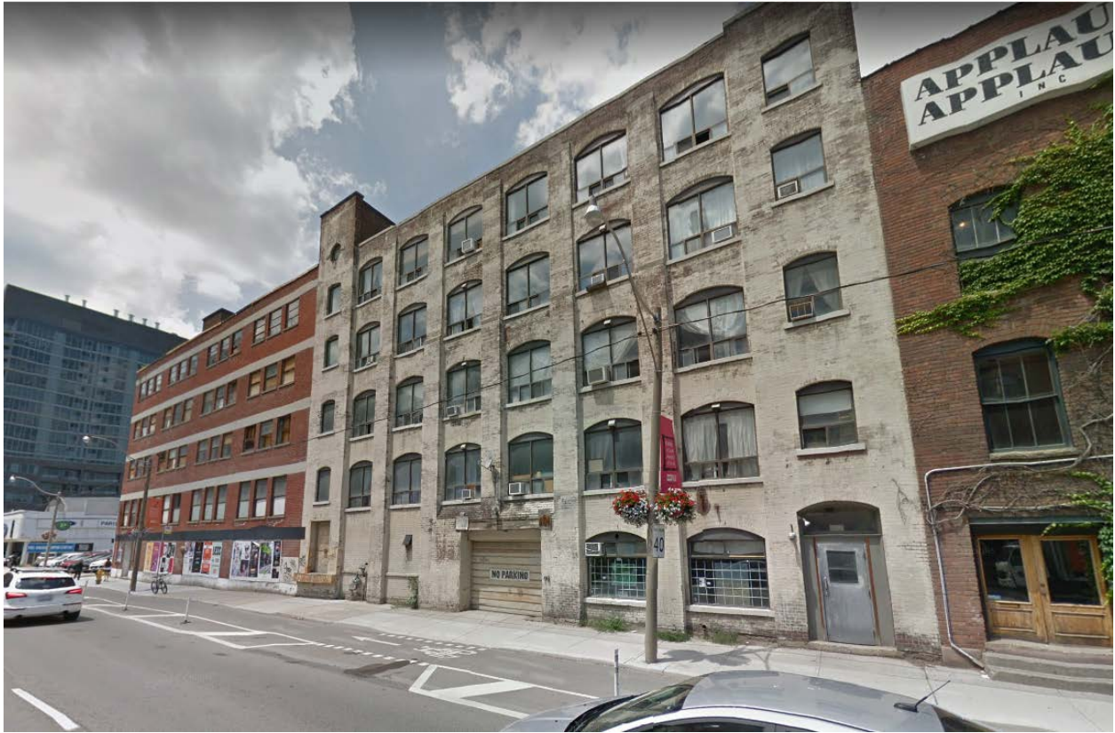
384 and 410 Richmond Street East - South Elevation
