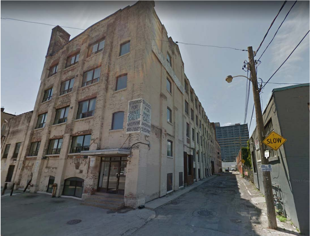
90 Ontario Street - East & North Elevations
