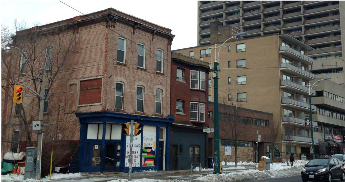
13. Photograph of the north-west corner of Spadina and Sussex avenues with the original building at 698 Spadina Avenue, the extended and altered building at 700 Spadina Avenue and the two-storey block at 704 Spadina Avenue dating from 1972 (HPS, 2016)
