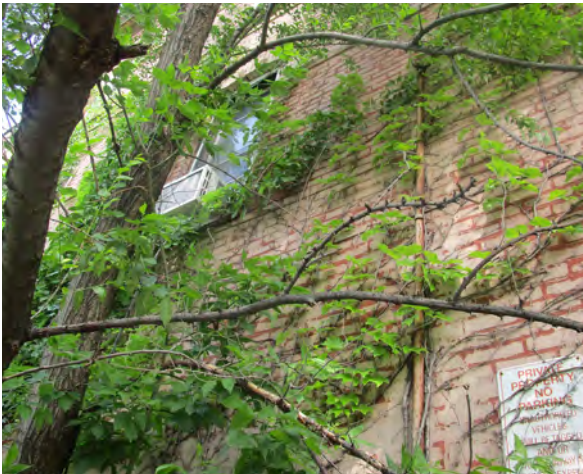
Fig.22: Vegetation obscuring building, South elevation.
