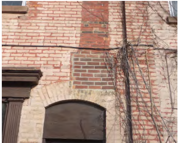
Fig.35: Brick infill cut into arch at South elevation.
