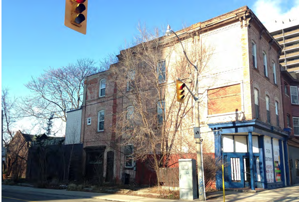
15. 698 Spadina Avenue showing the side (south elevation) with the lower rear wing, clapboard sunroom (1945) and the one-storey wall enclosing the property and linking with the rear gable roofed out building. (HPS, 2017)
