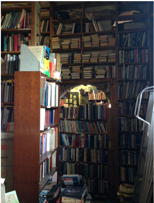
26. Interior of the bookstore, rear wing, looking towards the brick opening in the wall between the wing and the main building. (HPS, 2017)
