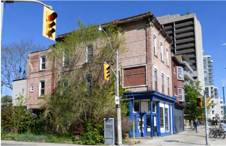
698 Spadina Avenue, southeast corner, 2016 (Source: ERA Architects).
