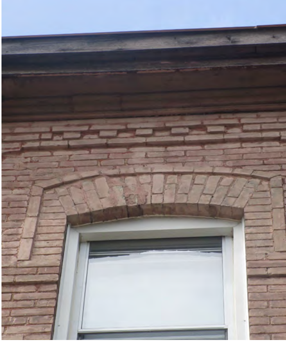
Fig.4: Parge repairs to segmental arch.
