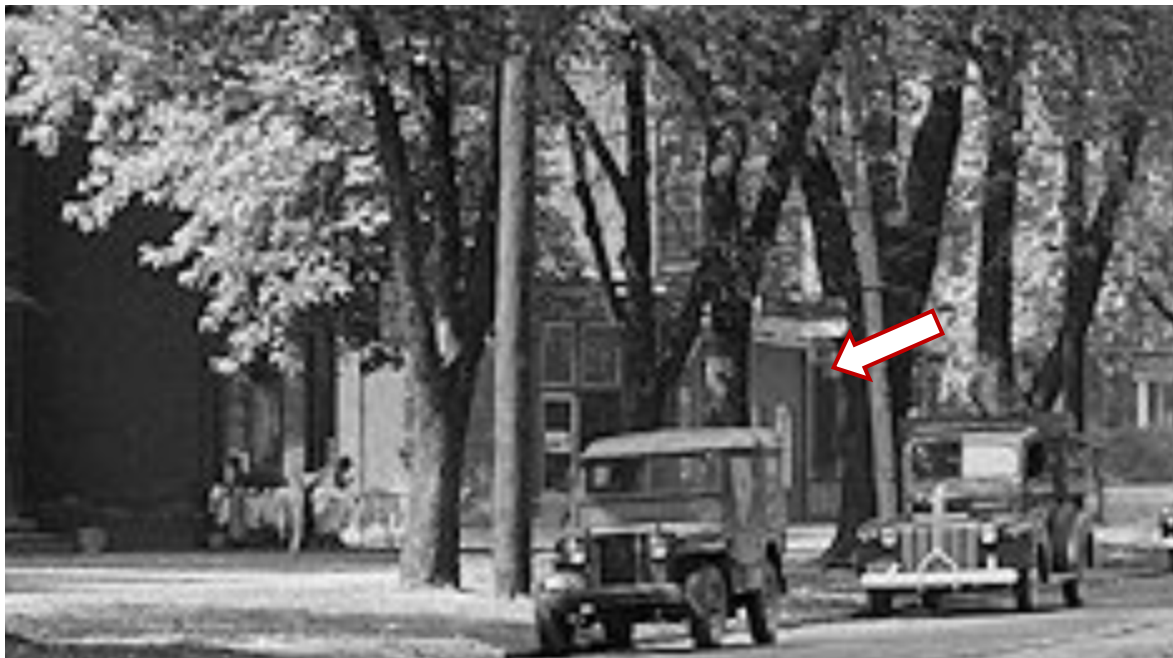
11. Detail of a photograph from 1945. Looking at the elevation of the building at 700 Spadina Avenue, between the two cars, the brick infill wall, the current window and the pilaster at the north end of the elevation can be seen. (CTA, Series 372, ss0058, it 1837)
