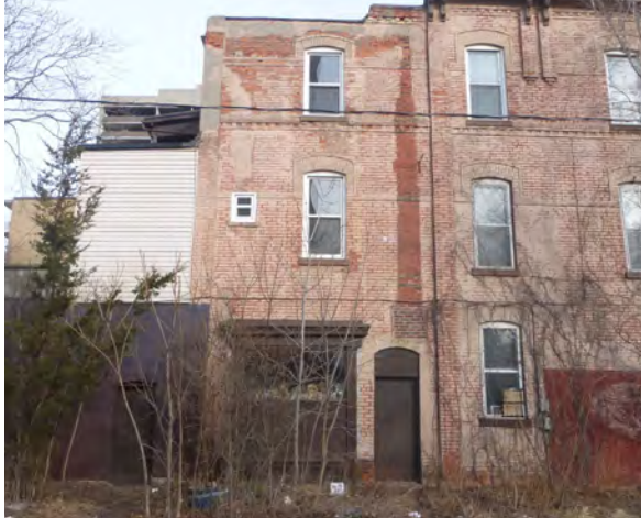
Fig.26: General condition of Western portion of South elevation.
