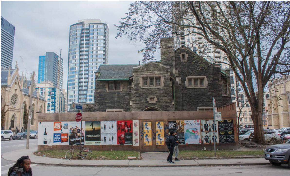
West Elevation of 51 Bond Street (ERA Architects Inc., 2017)
