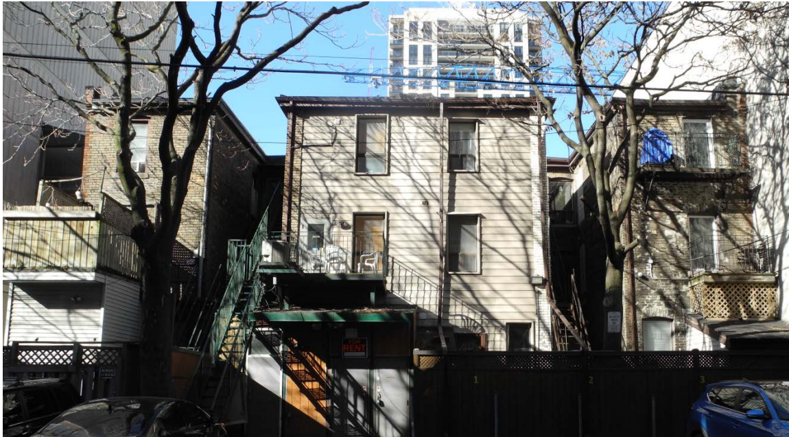
14. Photograph showing rear (east) elevations of the properties, showing the transition from red to buff brick (clad with siding at 39 and 41) and the two light wells shared between the four dwellings (CBCollective, 2018).
