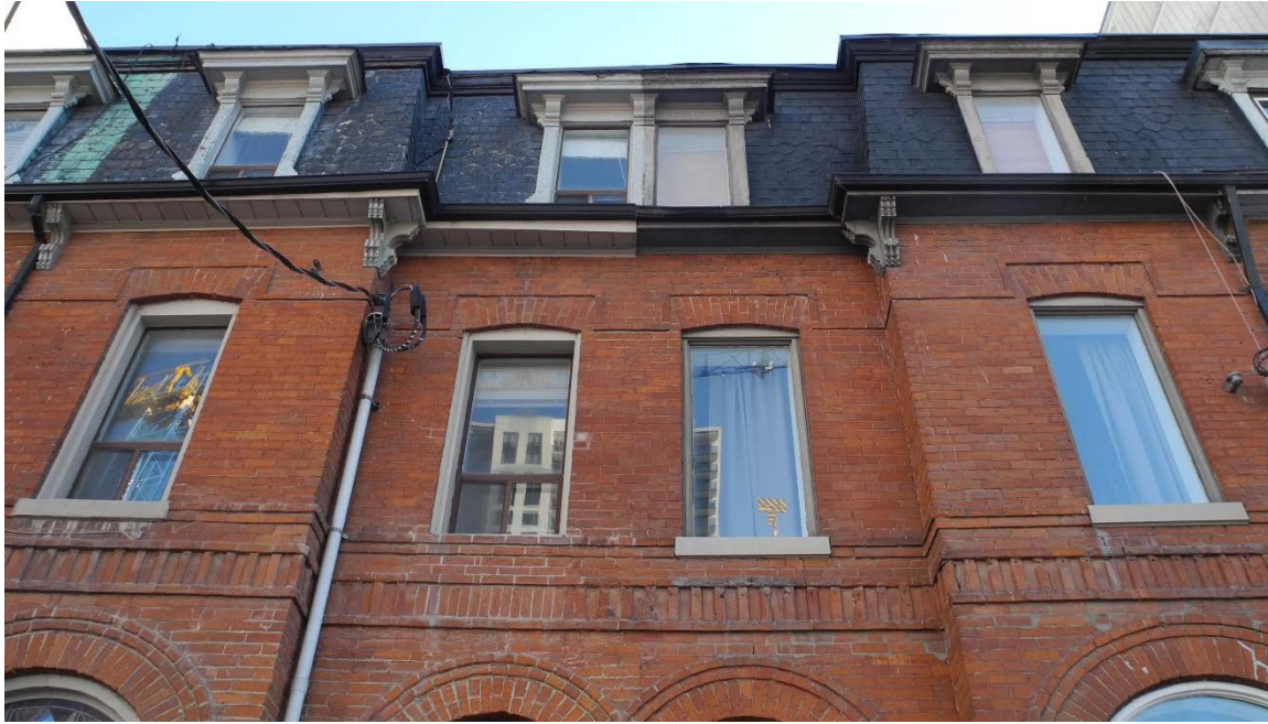
13. Photograph showing the decorative brick detailing at the first and second floor levels of the principal (west) elevations. Note the more recent tuck pointing of the brick at 39 Mutual, centre left (CB Collective, 2018).
