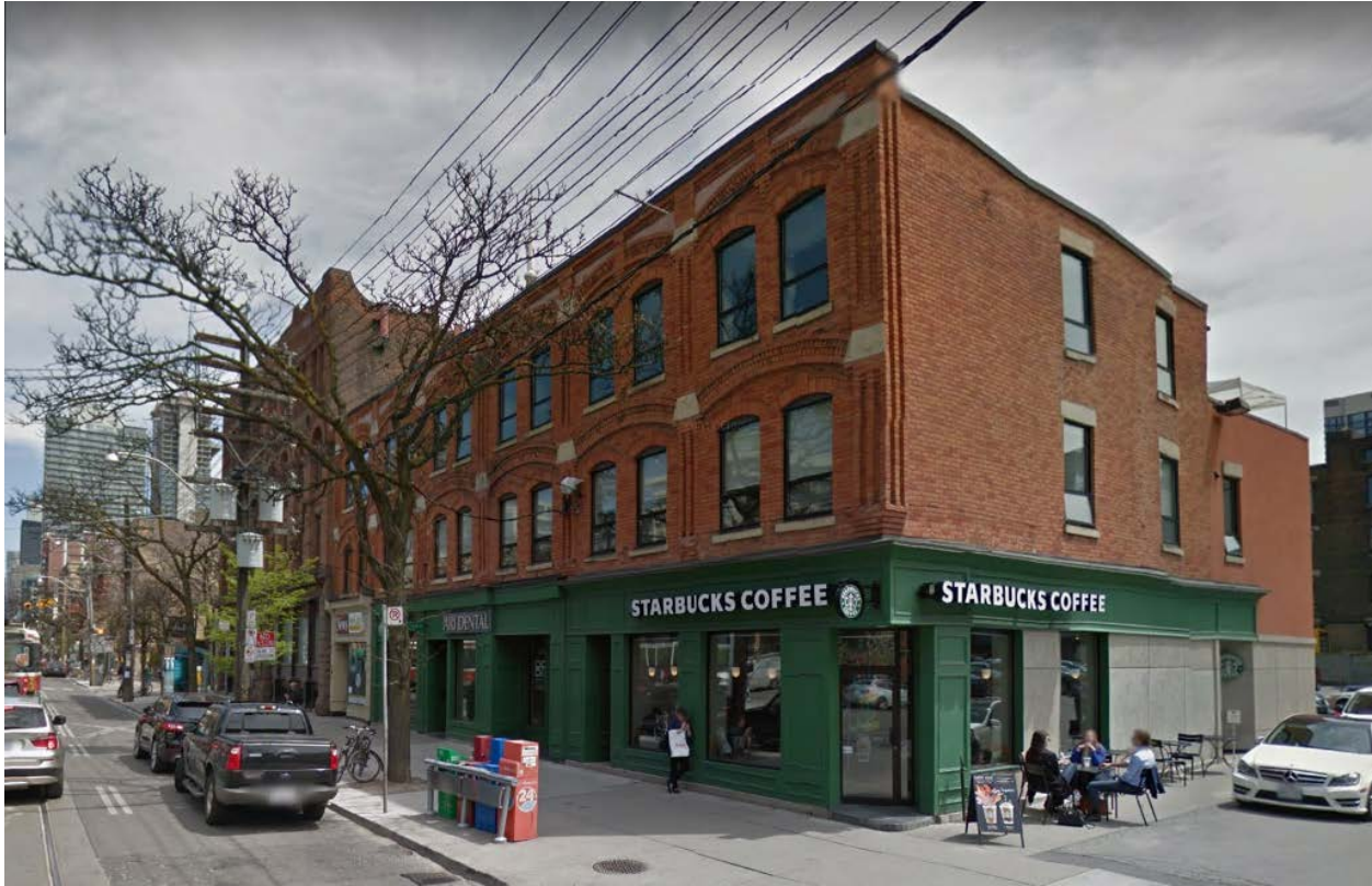
519-529 King Street West - north (King St) and west elevations
