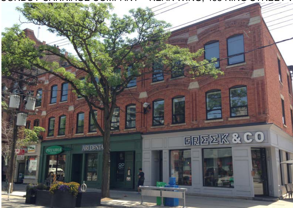
J. C. MUSSON BLOCK, 519-529 KING STREET WEST
