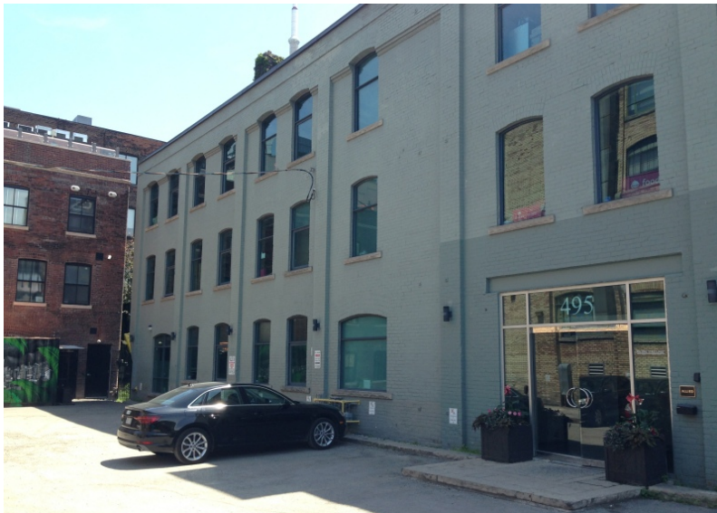
12. North elevation showing the entrance opening details and the relationship with the original Conboy building seen at the left of the photograph. (HPS, 2018)
