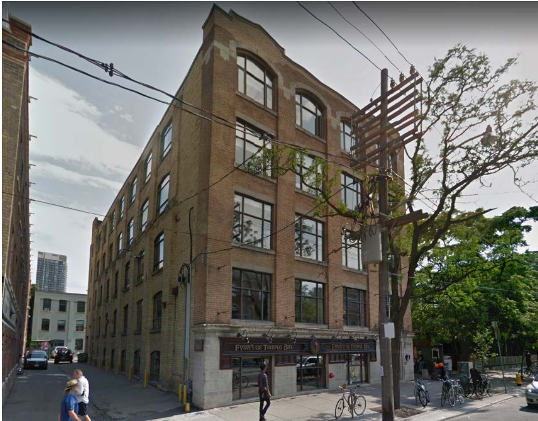
489 King Street West - north (King St) and east elevations
