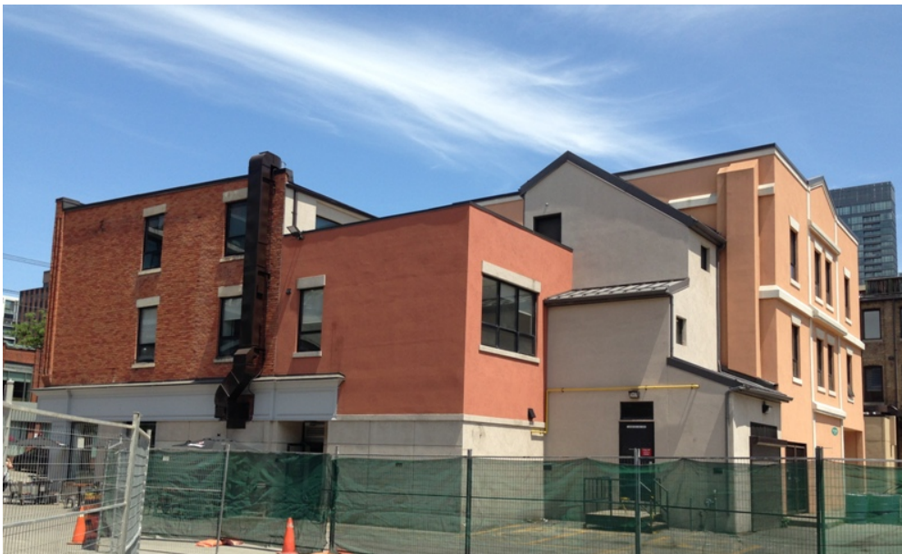
19. West Side and South Rear Elevations of 519-529 King Street West (HPS 2018)
