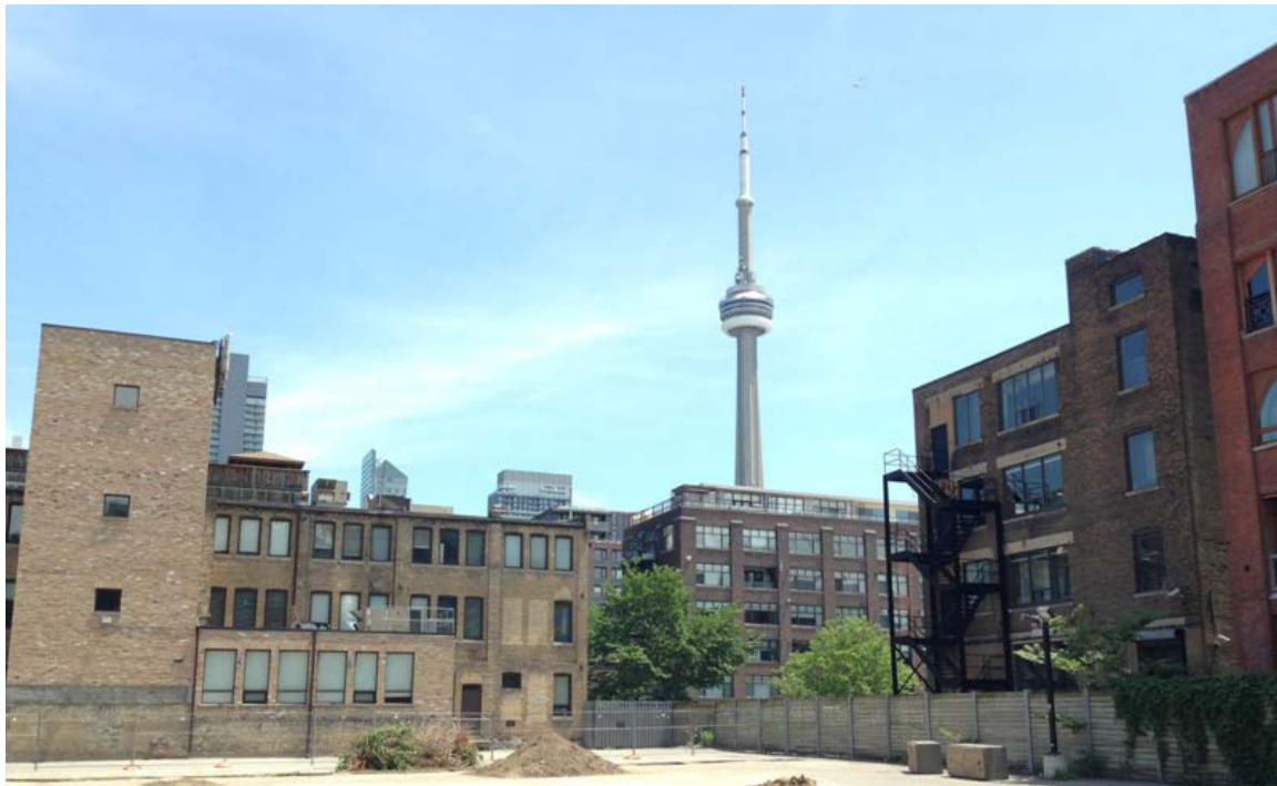
24. View east behind 519-529 King Street West towards Wellington Street West showing the context of warehouses (HPS, 2018)
