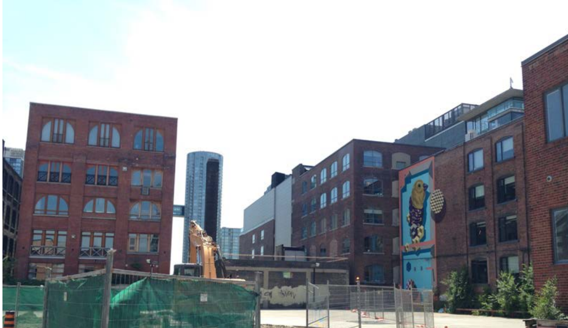
25. View towards Wellington Street West showing the context of warehouses (HPS, 2018)
