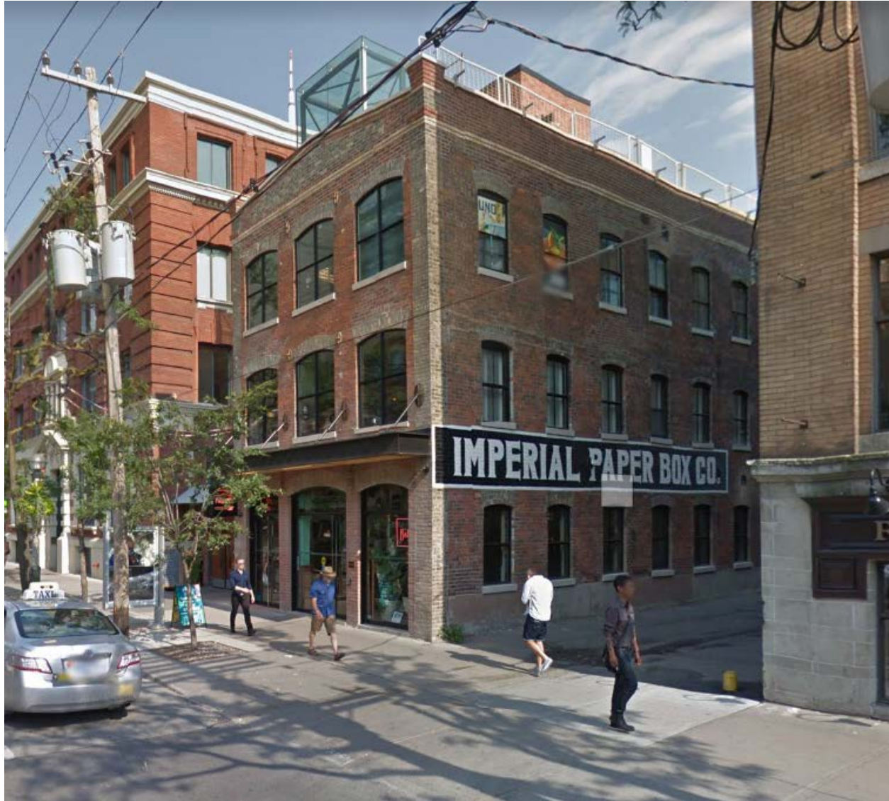
485 King Street West - north (King St) and west elevations
