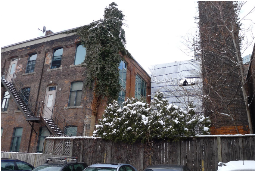
15. South and east elevations showing the alteration on the east elevation to add the pair of large curtain wall openings between the piers (HPS, 2016)
