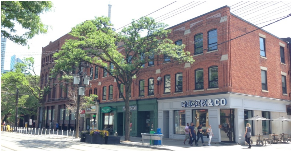
16. Photograph showing the principle north elevation and the side west elevation of the J C Musson Block at 519-529 King Street West (HPS, 2018)
