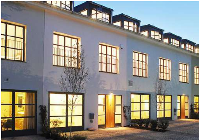
Figure 5.53: Mews-related residential units (London, UK)
