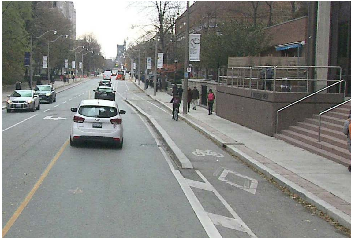
Example – Poured in Place Curb Wellesley Cycle Track
