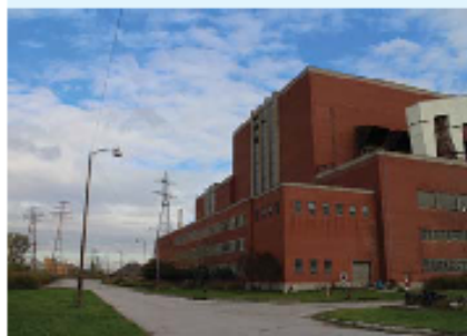
Hearn Generating Plant
