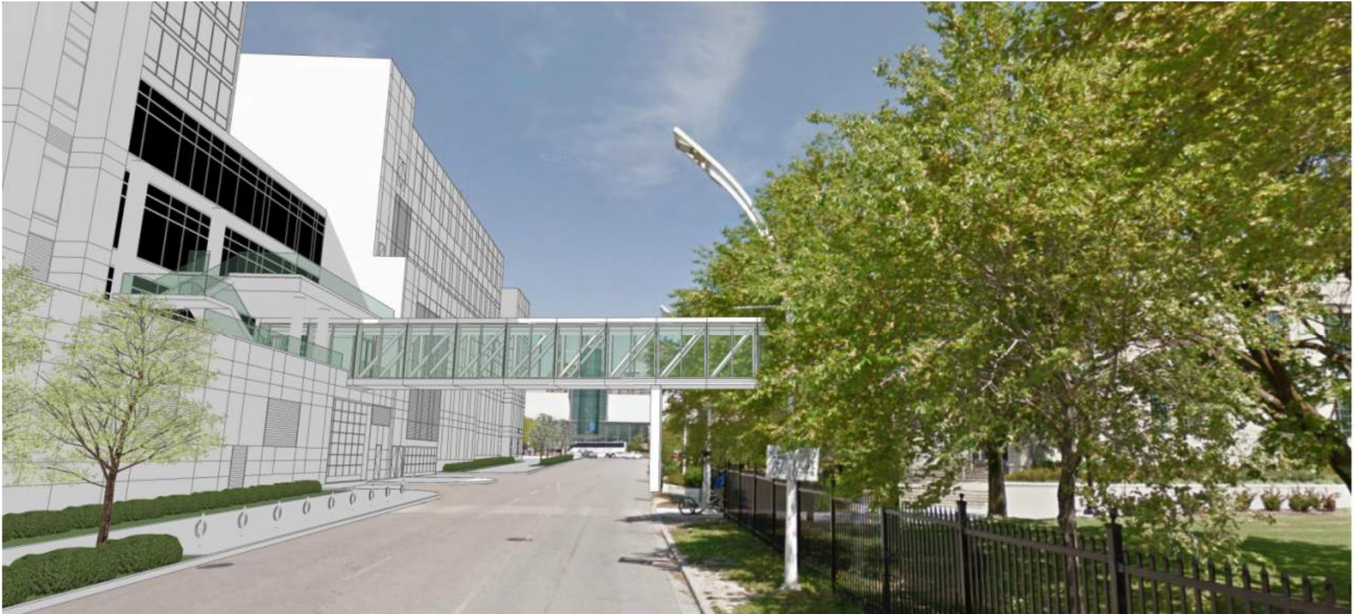
South Bridge view from Lakeshore Blvd.
