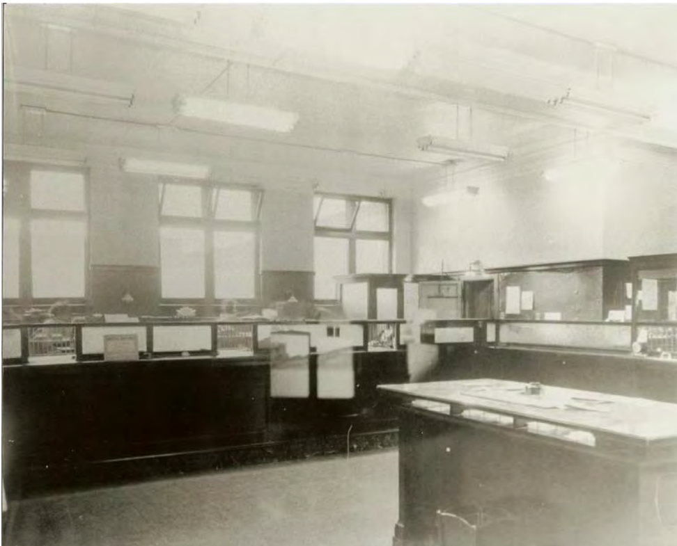
20. View of the CBC Banking Hall, 2896 Dundas Street West looking north towards the back of the building, no date but prior to the 1954 renovation and extension (WTJHS archives)
