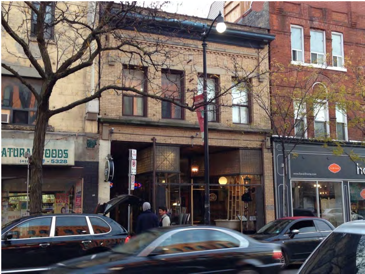
27. Block on the south side of Dundas Street West, as in Image 25, showing the late 19th and early 20th-century mixed use buildings with some original shop fronts and details (HPS 2017)
