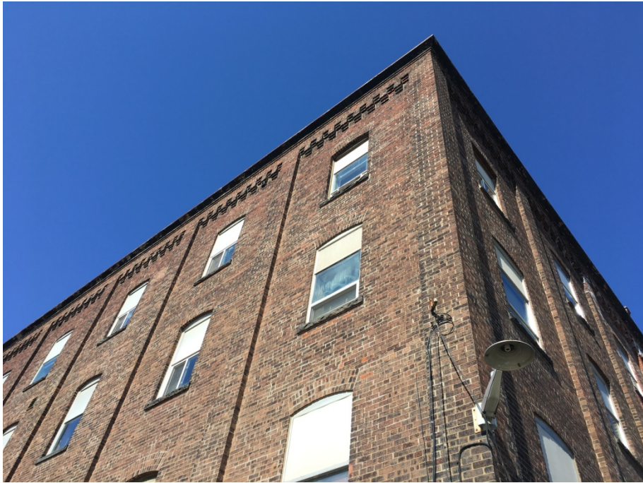
South-West Corner of 30 Powerhouse
