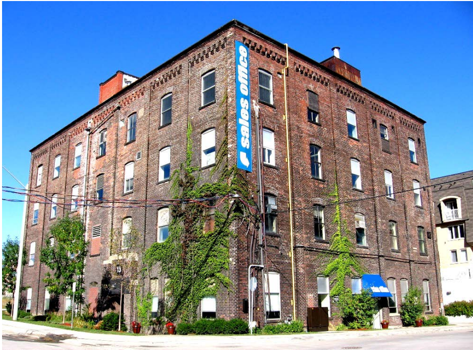
View Looking North-East from Foundry Avenue (2011)
