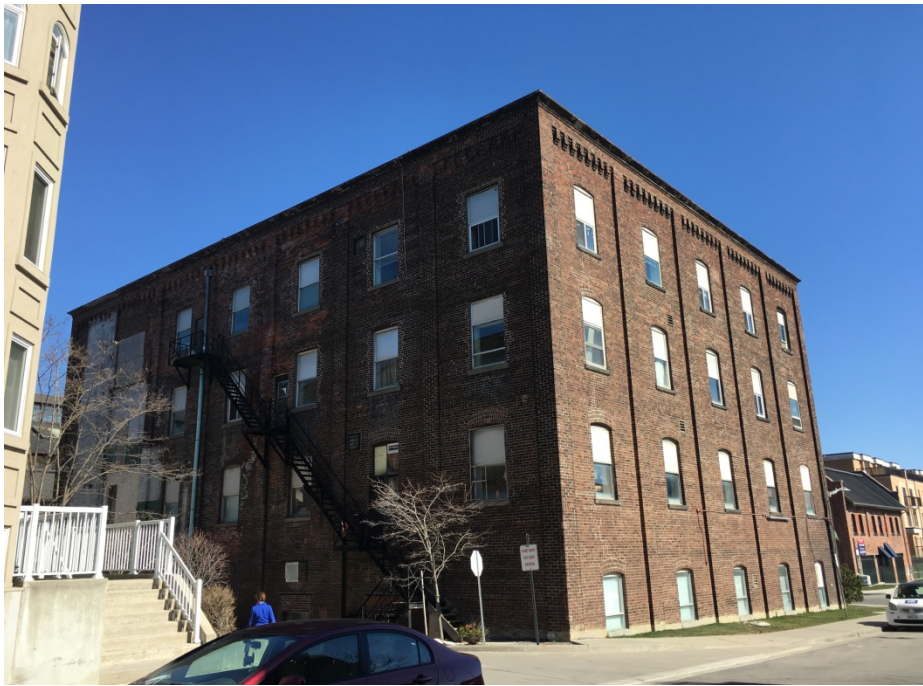
View Looking South-West from Foundry Avenue (2018)
