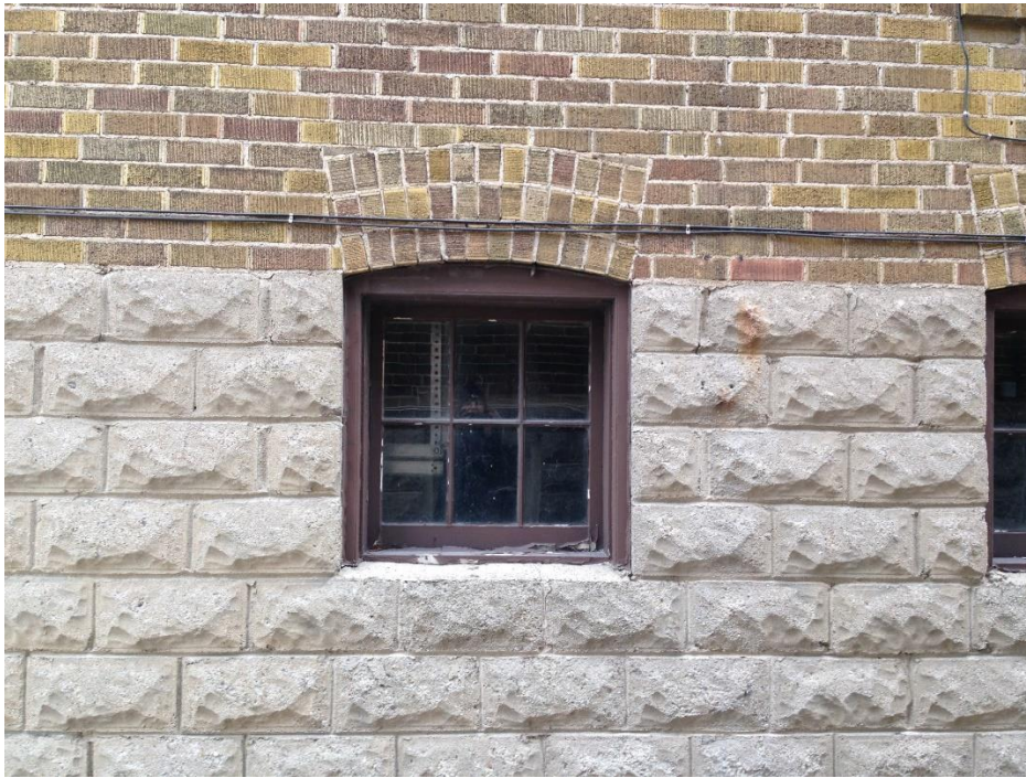
12. Side wall and window at 1783 Bayview Avenue showing the use of rusticated concrete block also used at the building at 1755 Bayview Avenue and the other eight apartment blocks in the sequence. (HPS, 2017)
