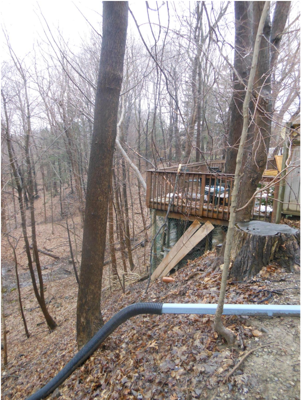
Photo 3. Photograph illustrating relationship between existing rear deck and the ravine. Photo taken March 07, 2017 by RNFP Staff.
