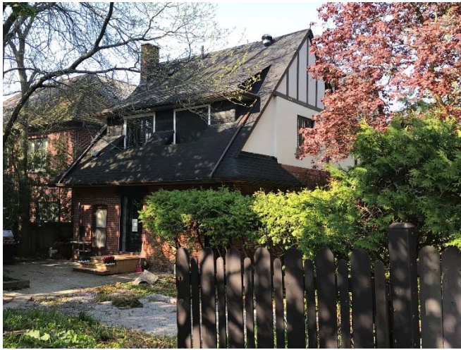
12. Left: Albert E. Knox House, east elevation showing the double shed dormers on the second storey (HPS, 2018)
