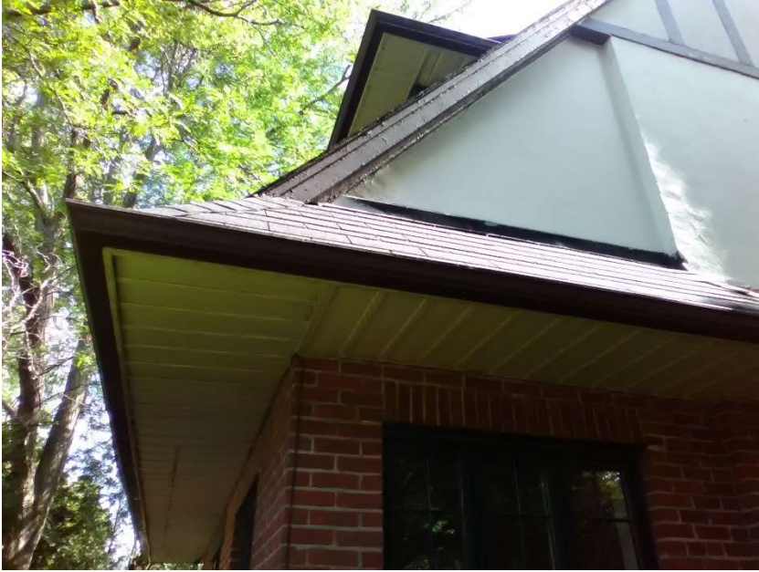
Figure 3: Modern Aluminum Soffits throughout
