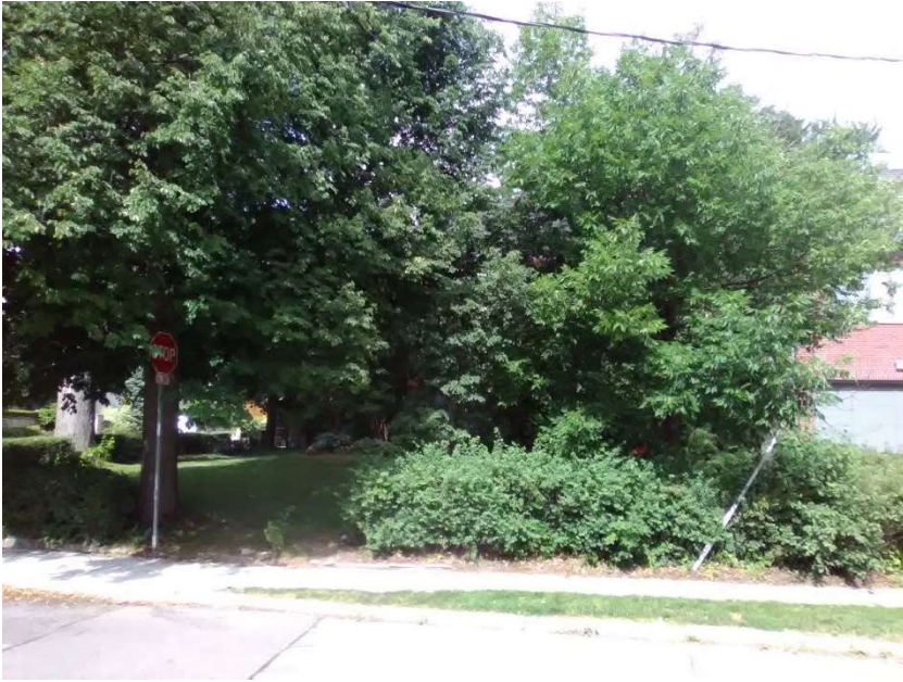
Figure 4: View of the West Elevation from the Street
