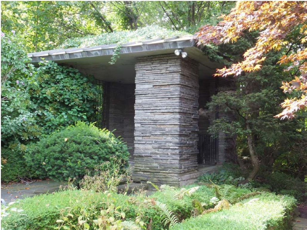
7 Dale Avenue- teahouse structure in rear yard
