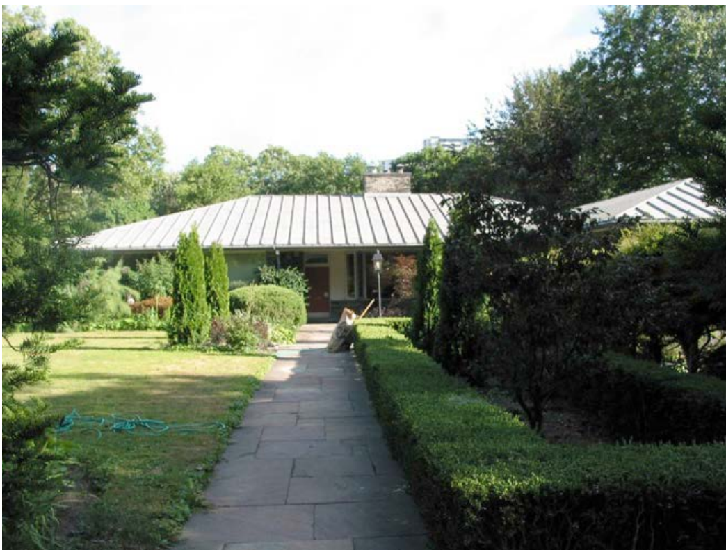
7 Dale Avenue- north view of L-shape house with landscaped forecourt
