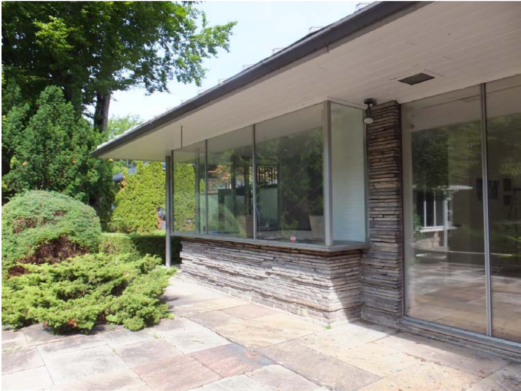
7 Dale Avenue- view of partial south elevation
