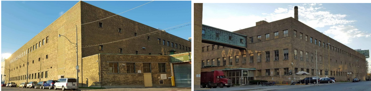
6b and 6c. Warehouse, with the east elevation and part of the north elevation (left), and the west elevation and part of the north elevation (right)
