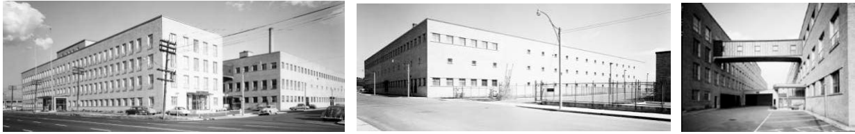
4a, 4b and 4c. LCBO office building and warehouse from the north (left), the warehouse from the south (centre), and bridge connecting the office building and warehouse (right) in 1955
