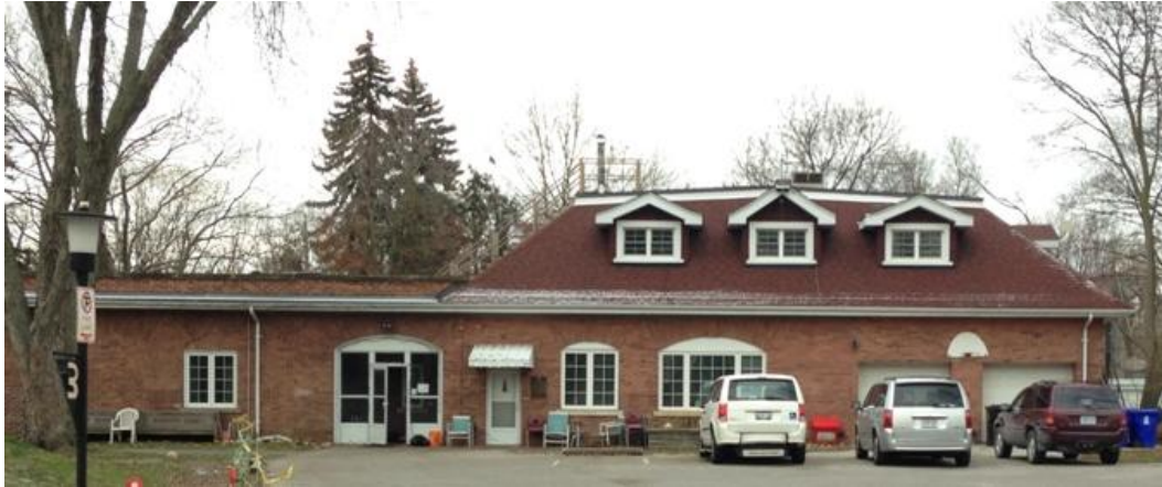
10. East Elevation of the Coach House (HPS, 2017)
