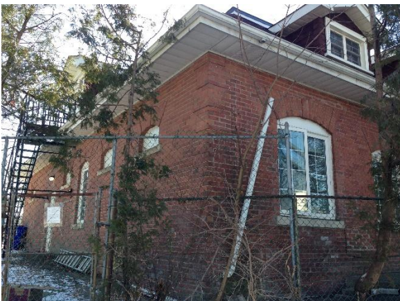
15. West and North Elevation of the Coach House showing the windows and the brick detail (HPS, 2018)
