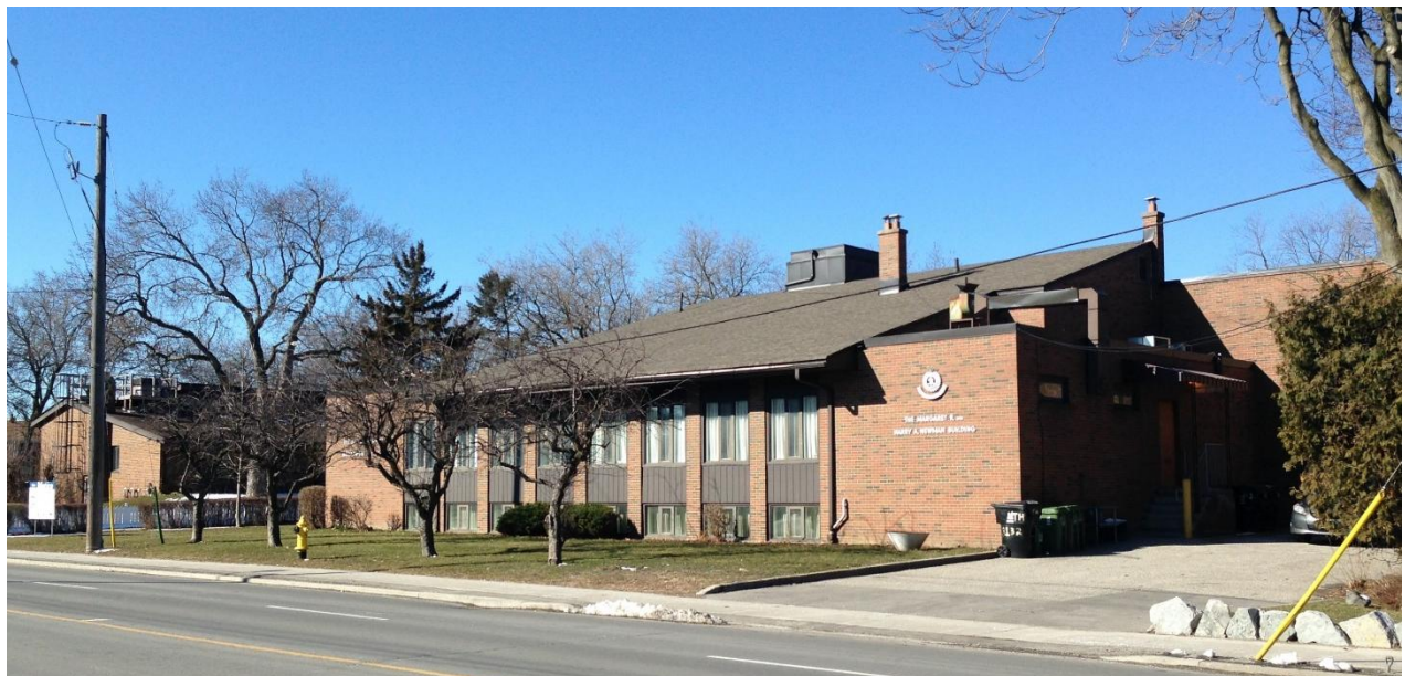
Photograph of the Salvation Army Broadview Village, with the Margaret R. and Harry A. Newman Building (right), principal (east) elevation, and one of the cottages on the far left showing a side (east) elevation (HPS, 2018)
