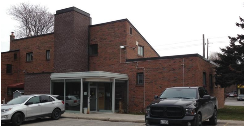
29-32. Photographs showing the principal east and side (south) elevations, the Salvation Army insignia above the building's name acknowledging the Newman's (top), the rear west elevation (middle) and the new entry and elevator addition (2010) (below) (HPS, 2017-2018)
