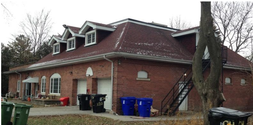
11. East and North Elevations of the Coach House (HPS, 2017)
