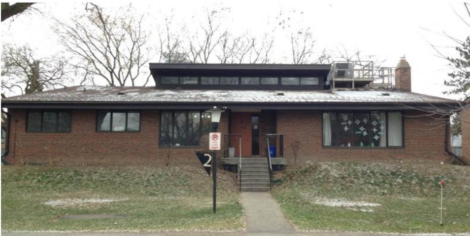
19. North (Principal) elevation of a typical cottage. (HPS, 2017)
