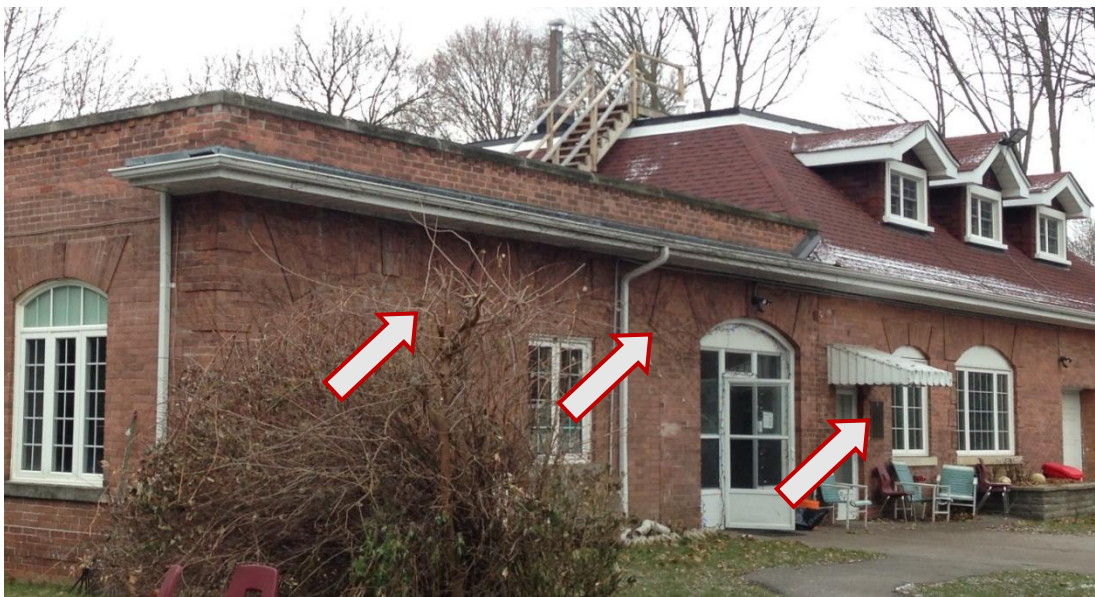
12. West and East Elevation, Coach House. The arrows indicate the brick arches and voussoirs which remain following the 1961 brick infills. Next to the canopy the quins indicate the edge of the original coach house before the south wings was added (HPS, 2017)
