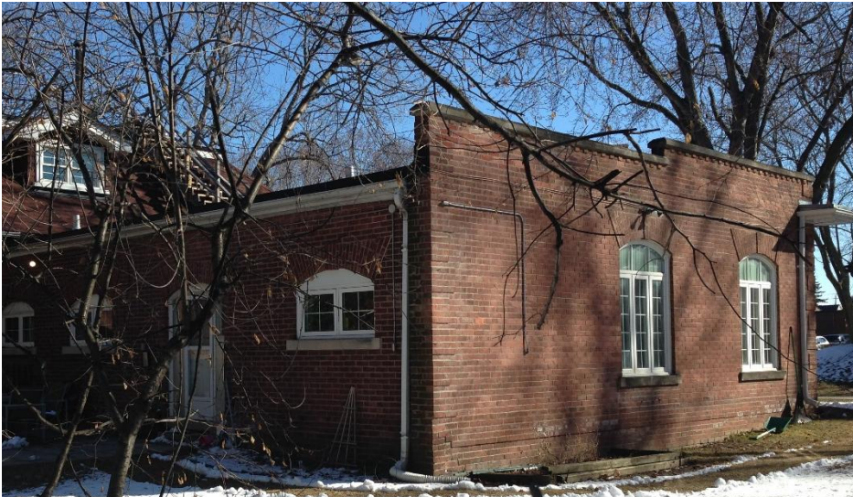
14. South and West elevations showing the brick relief (HPS, 2018)
