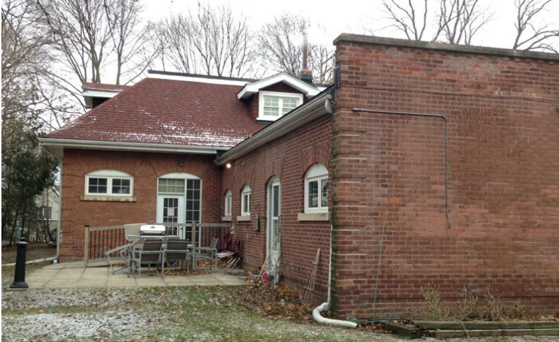
13. South and West elevations showing the various windows related to the coach house function and the 1961 alterations in the corner (HPS, 2017)
